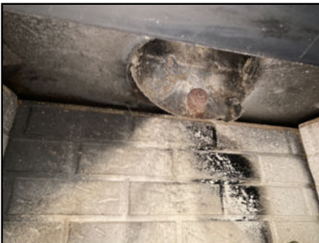
Damper door is stuck - needs to be serviced
