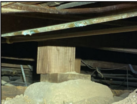
Posts off centered and not aligned over concrete piers - recommend brackets for added support
