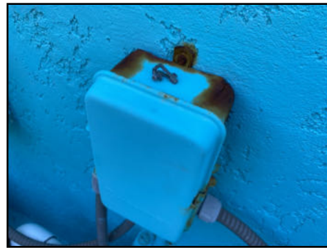
Corroded junction box - needs to be serviced
