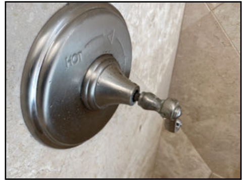
Shower fixture handle(s) loose - needs to be serviced
