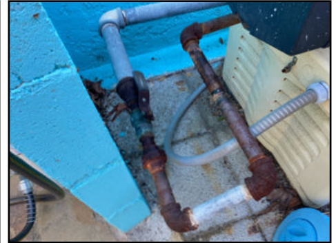
Corroded fuel gas piping - needs to be serviced
