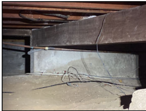
Unsecured wiring - needs to be serviced - All wiring should be properly secured to the framing.
