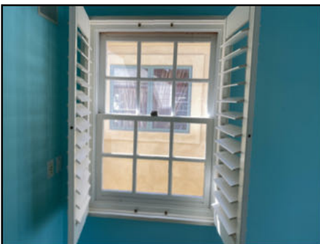
Did not open properly - needs to be serviced - Master & Upstairs South Bedrooms
