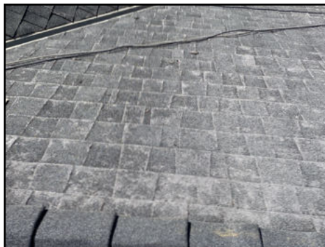
Shingles exhibited extensive/abnormal granule loss - needs to be serviced/evaluated by a roofer
