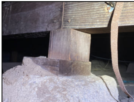
Posts off centered and not aligned over concrete piers - recommend brackets for added support
