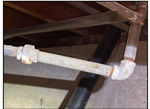
Corrosion present on gas piping - needs to be serviced
