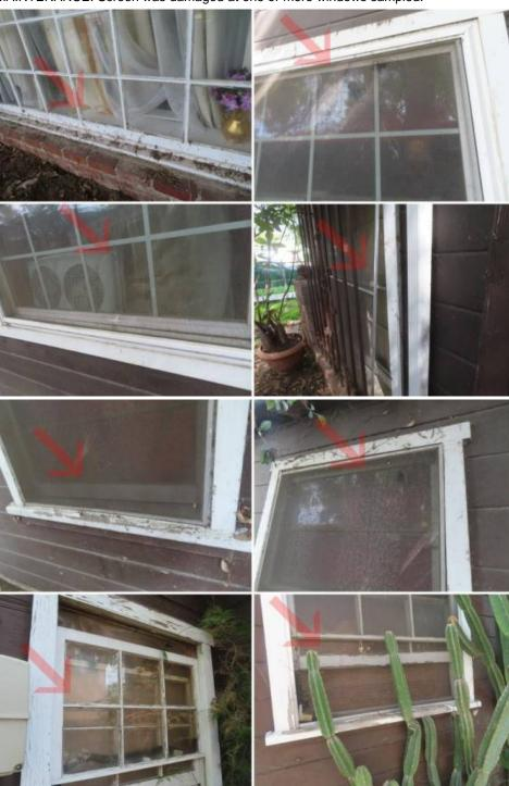
time to protect the wood from further deterioration and to enhance its appearance. MAINTENANCE: Screen was damaged at one or more windows sampled.
