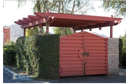
Figure 11. Trash enclosures with architectural screening elements.
