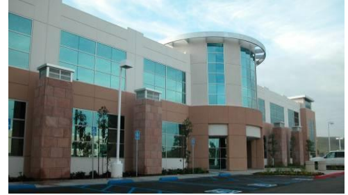
Figure 20. Incorporation of vertical offsets and material changes.
