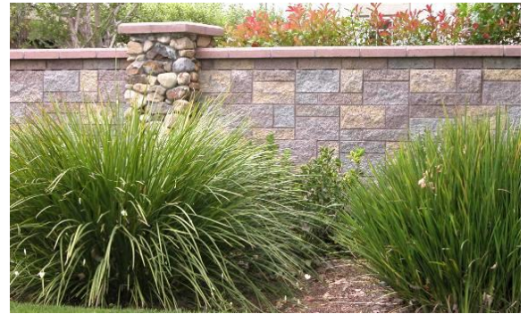
Figure 40. Wall incorporates pilasters and cap.
