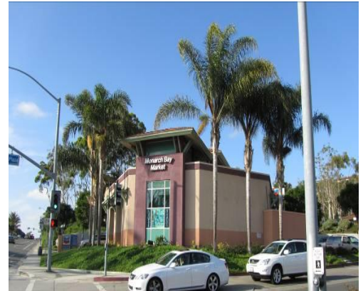
Figure 96. Corner landscaping element.
