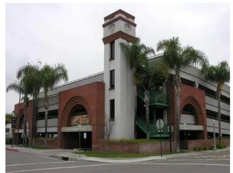
Figure 94. Paving differentiates between pedestrian and vehicular entries.
