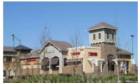
Figure 64. Exterior finish materials.
