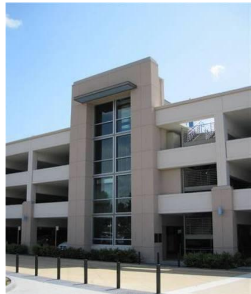
Figure 95. Glass-back elevator cab and shaft.
