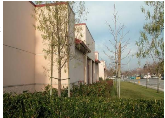
Figure 90. Articulated wall of mini-storage facility.
