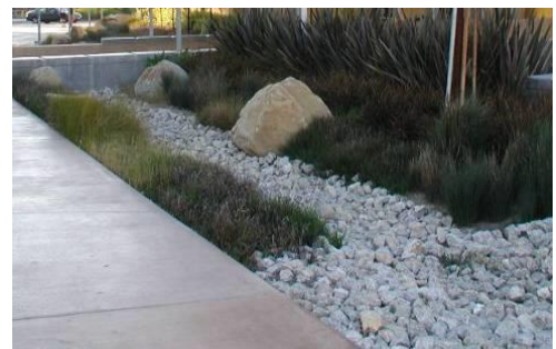
Figure 33. On site water filtration.
