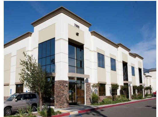
Figure 83. Awnings articulate entries to tenant spaces.
