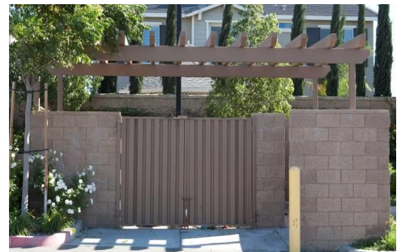
Figure 76. Trash enclosures with architectural screening elements.
