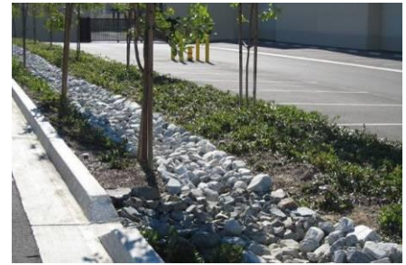
Figure 17. On-site stormwater capture system.
