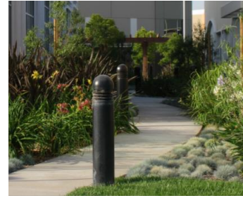
Figure 45. Bollard lighting along pedestrian walkway.
