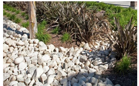
Figure 79. On-site stormwater capture system.
