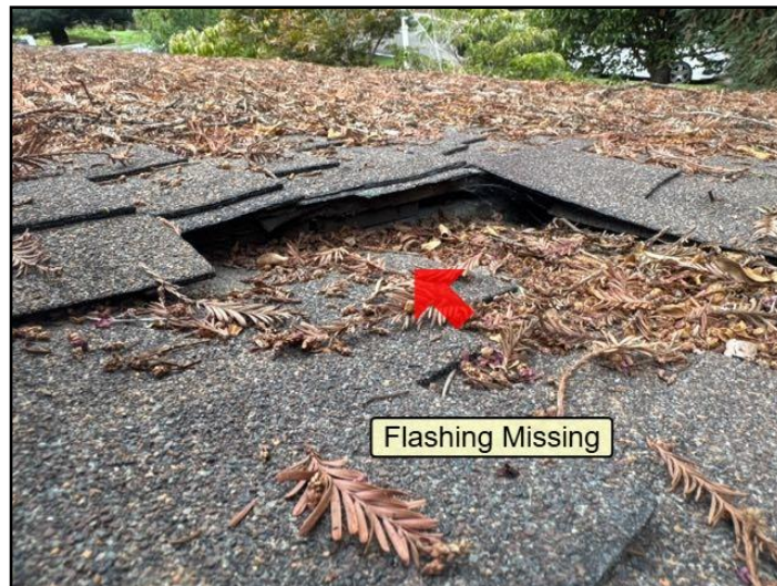
8. Flashing missing
