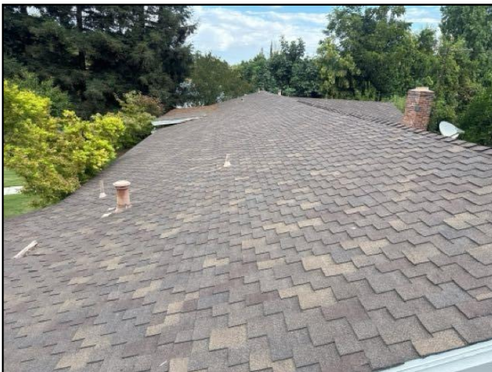
1. Asphalt shingles
