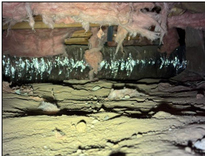
50. Ducts and registers
