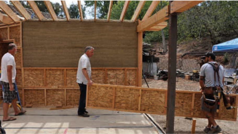
Taking off forms and exposing hempwall
