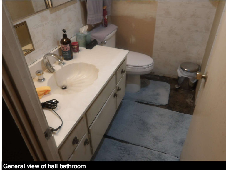
General view of hall bathroom
