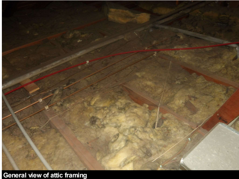
General view of attic framing
