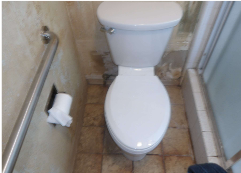
General view of toilet
