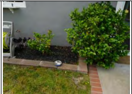
Rear elevation planter terminates against stucco finish
