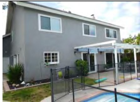
Overview of rear elevation
