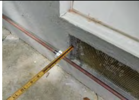
Overview of stucco termination at concrete hardscape at right side elevation
