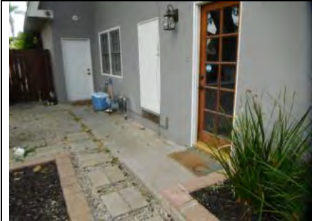
Overview of stucco termination at concrete hardscape at right side elevation
