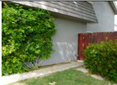
Right side elevation, planter grade terminates against stucco
