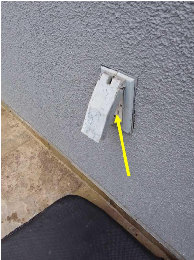
The outlets are functional and include ground-fault protection.
