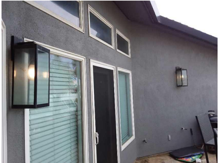
The lights outside the doors of the residence are functional.
