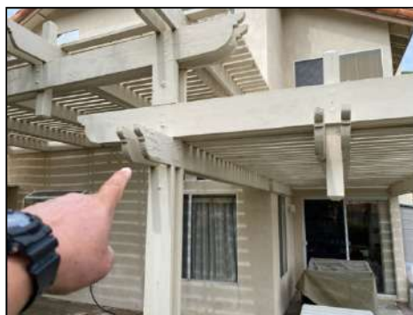
Wood deterioration observed - consult termite report
