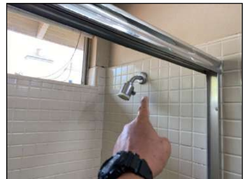
Shower arm faceplate is loose at the wall - recommend securing and sealing this area
