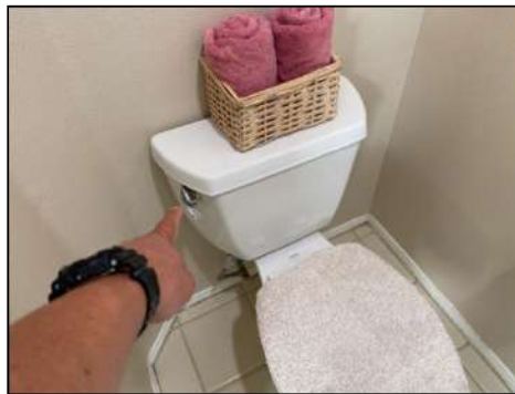
Toilet flush valve was leaking - needs to be serviced
