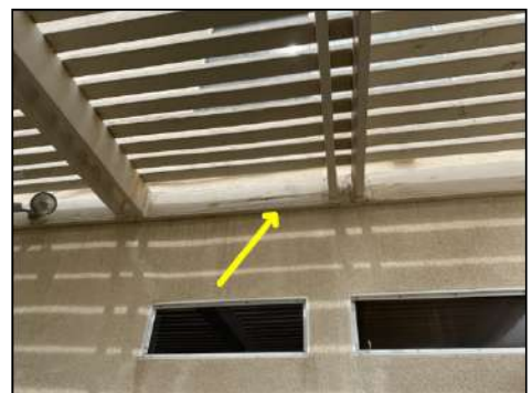
Wood deterioration observed - consult termite report
