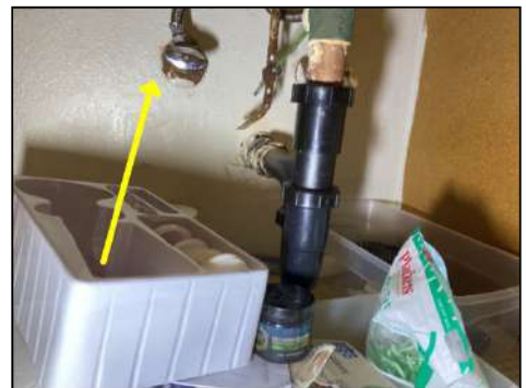
Corrosion is present at plumbing areas - this is a sign of slow leaking and should be further evaluated by a plumber
