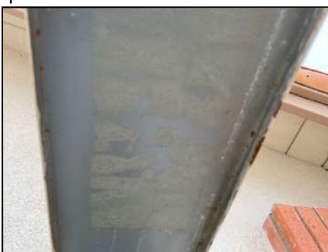
Panel rating label not legible or missing - main amp rating is unknown
