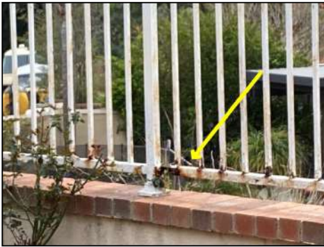
Rust/rust damage at metal fence materials - needs to be serviced
