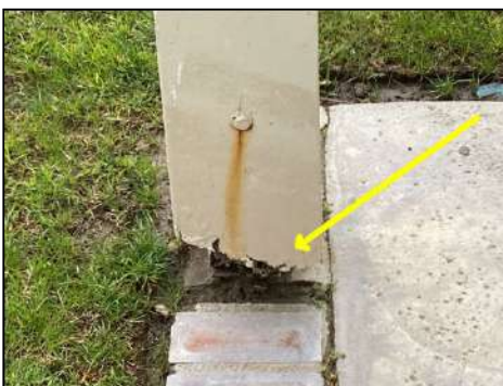
Wood deterioration observed - consult termite report
