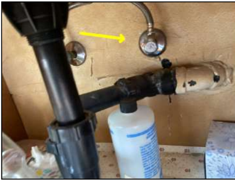
Corrosion is present at plumbing areas - this is a sign of slow leaking and should be further evaluated by a plumber
