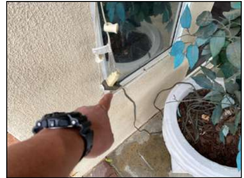
Using extension cord for power - recommend servicing
