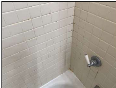
Surface microbial growth/irregular staining is present in areas on nonporous surfaces - recommend cleaning and sealing materials regularly
