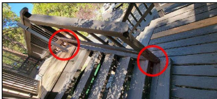
33. Rot or insect damage
