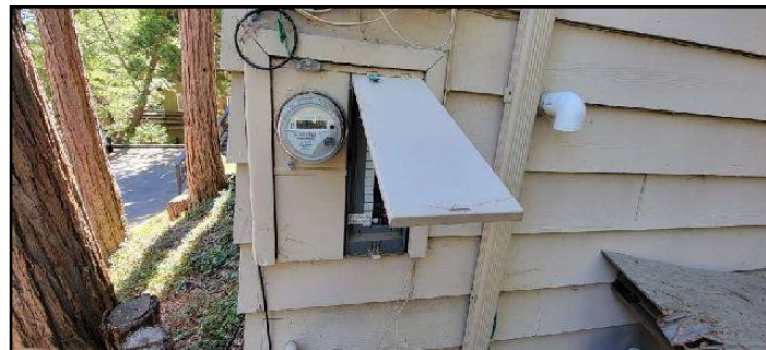
42. Breakers - exterior wall
