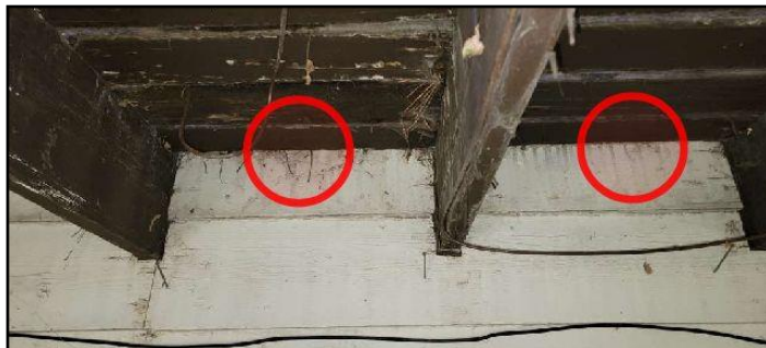
31. Missing flashing at deck connection
