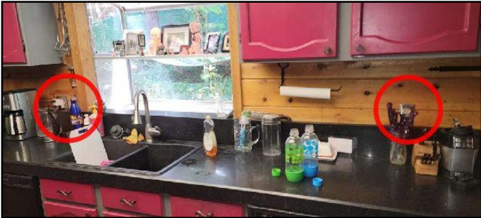
45. GFCI/GFI needed (Ground Fault Circuit...
