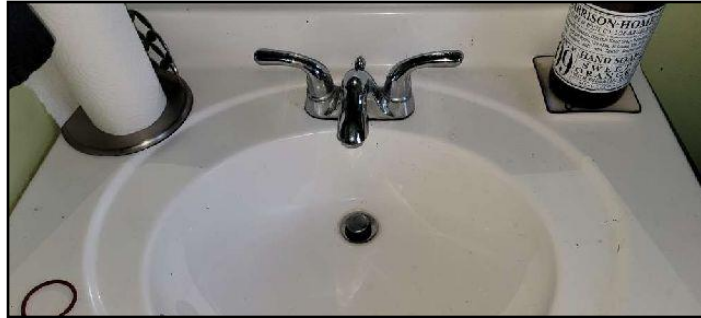
70. Drain stop ineffective
