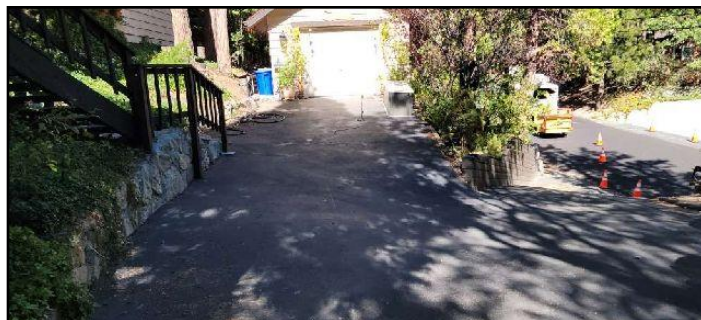
7. Away from building
