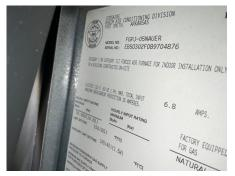
81: TYPE: Gas, forced air, furnace present. Furnace is rated for MAX Input 50,000 BTUs.
