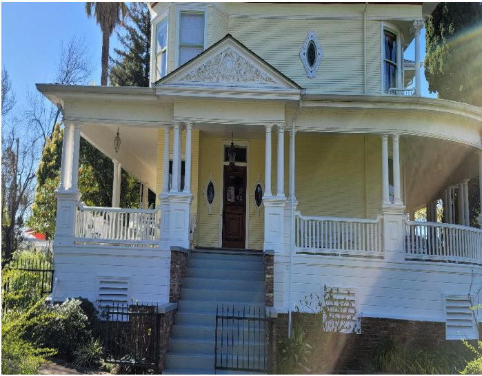
- Front of the structure.
