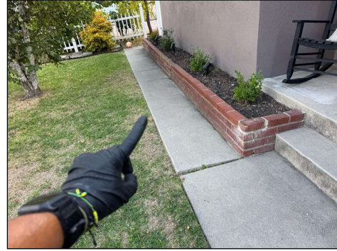
Walkway displacement/uplifted/uneven areas – potential tripping hazard – service recommended
