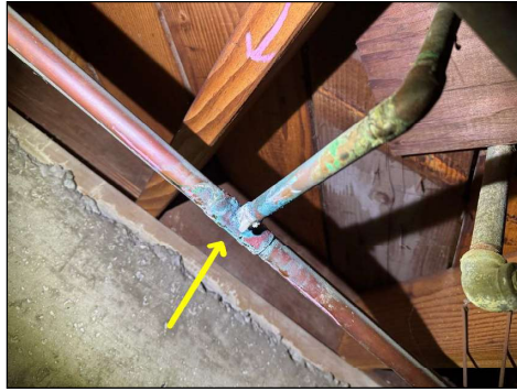
Copper tubing discolored – electrolysis present in areas - visible leaking in one area - service recommended
