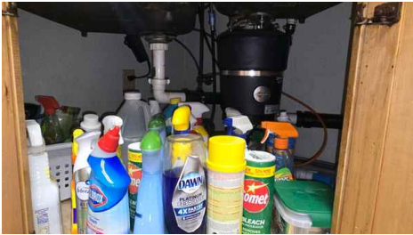
Sink, Faucets, & Drains: Below Sink
