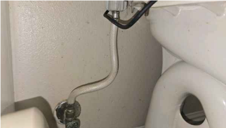
Sink/Faucet/Drains/Supply: Angle Toilet: Angle Stops Stops
