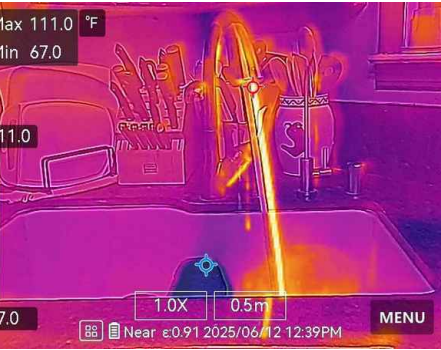
Garbage Disposal: Brand ISE
