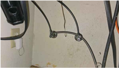
Sink, Faucets, & Drains: Angle Stops
