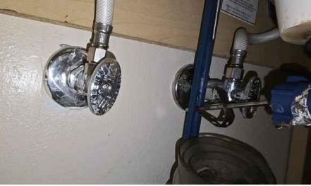
Sink/Faucet/Drains/Supply: Angle Toilet: Angle Stops Stops
