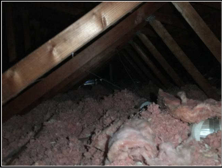
View of attic.
