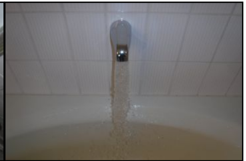
Fixture loose/gapped at wall - recommend sealing all fixtures where attachments meet the wall to ensure that moisture does not enter the wall
