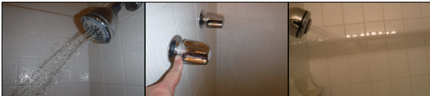
Caulk maintenance needed at wall to fixture juncture
