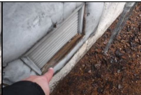
Deteriorated wood present - enclosure door
