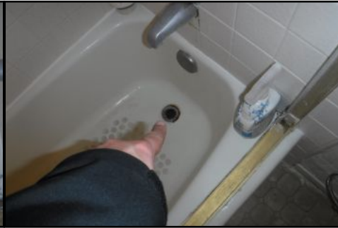
Drain stopper missing - needs to be serviced - downstairs
