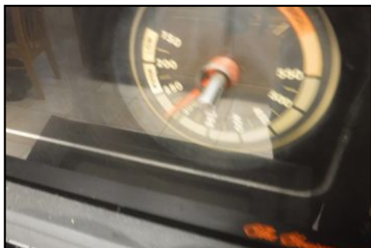
Temperature control knob missing - needs to be serviced
