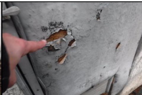
Deteriorated wood present - enclosure door
