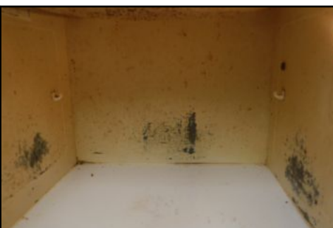
Chipped/rusted/exposed metal inside at walls - needs to be serviced
