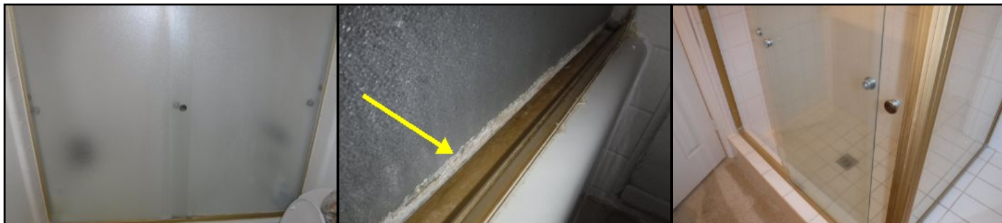
Corrosion present in areas - signs of wear and moisture accumulation
