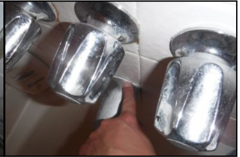
Fixture loose/gapped at wall - recommend sealing all fixtures where attachments meet the wall to ensure that moisture does not enter the wall
