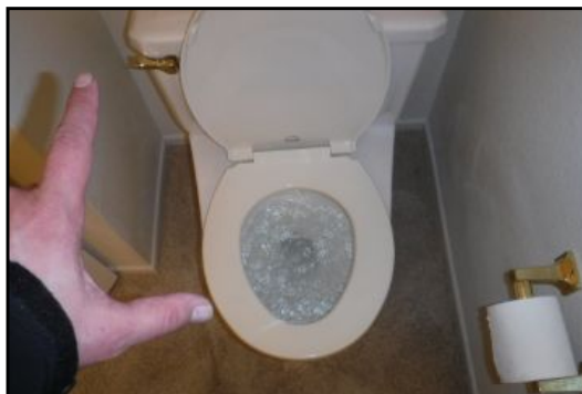
Toilet slightly loose- recommend tightening to prevent water damage - master
