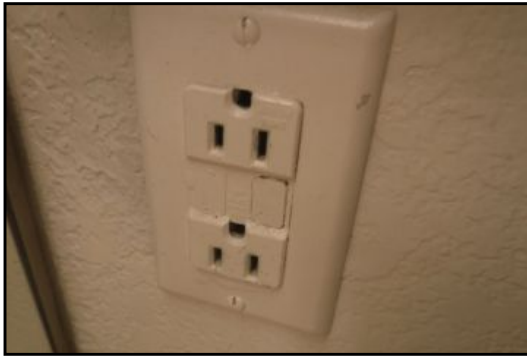
Worn/loose GFCI outlet - needs to be serviced
