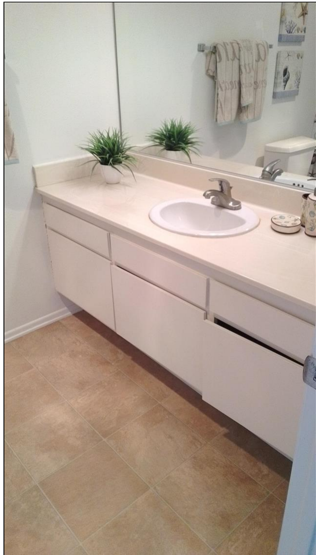
4.5 Item 2(Picture) 2nd floor primary bedroom bathroom base cabinets
