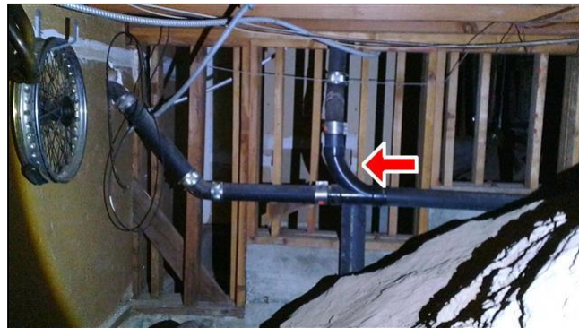
6.5 Item 5(Picture) Cast iron/ABS replacement, drain lines
