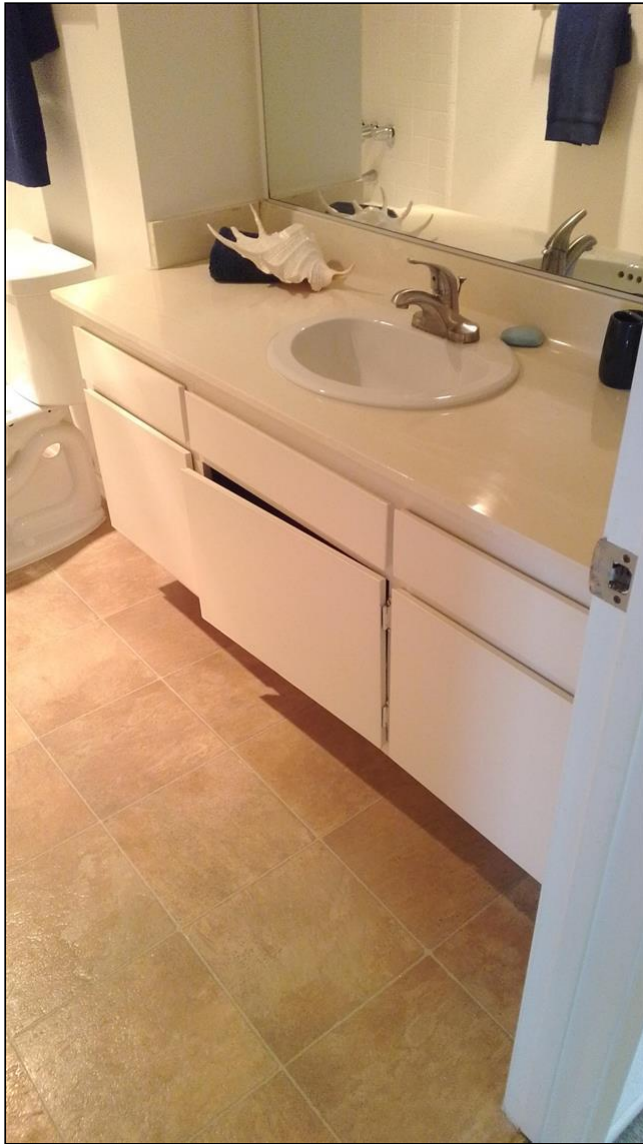
4.5 Item 1(Picture) 2nd floor hall bathroom, base cabinets
