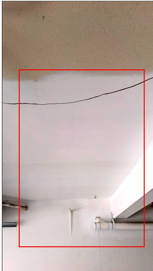
3.1 Item 1(Picture) Garage ceiling repairs
