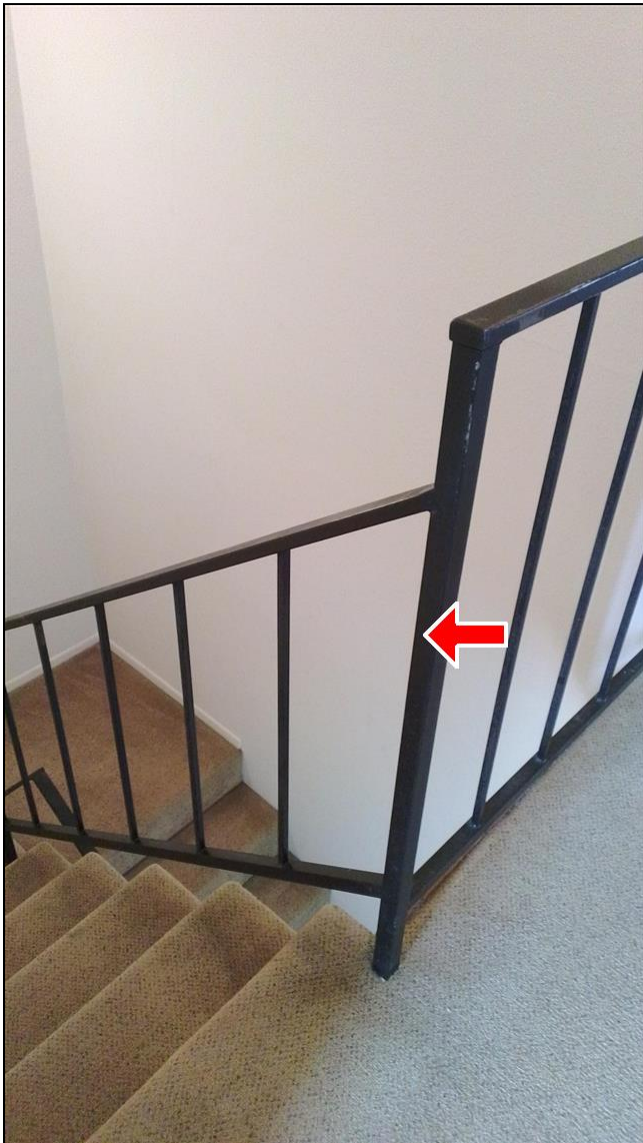
4.4 Item 1(Picture) Stairwell railing
