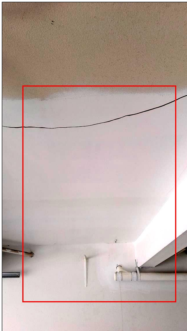
3.1 Item 1(Picture) Garage ceiling repairs
