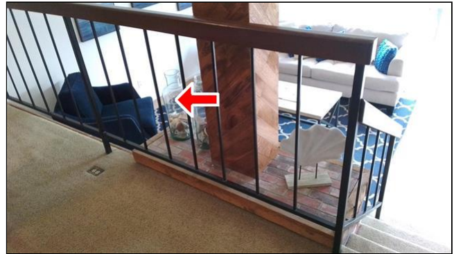
4.4 Item 2(Picture) Guard railing
