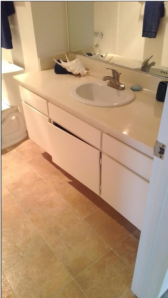
4.5 Item 1(Picture) 2nd floor hall bathroom, base cabinets
