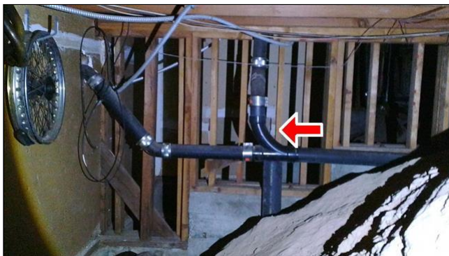
6.5 Item 5(Picture) Cast iron/ABS replacement, drain lines
