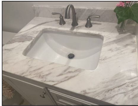
Caulk maintenance needed at backsplash to countertop joint - needs to be serviced
