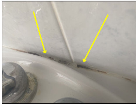
Caulk maintenance needed at backsplash to countertop joint - needs to be serviced
