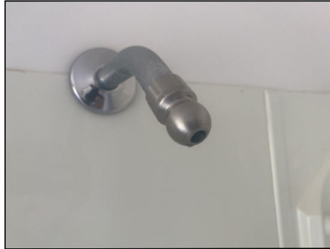
Shower head attachments missing - needs to be serviced
