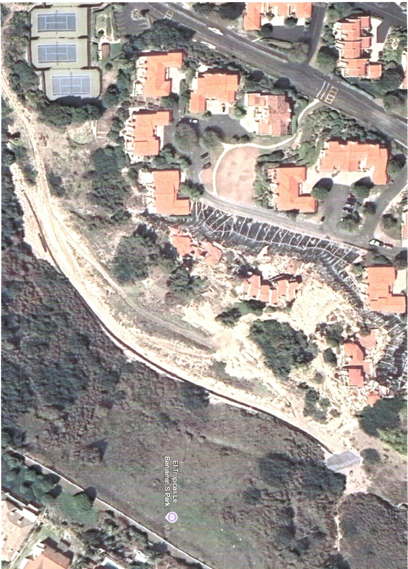
The Berm & Water Drainage Pipe
