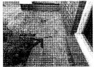
Moss is visible on the surface of the front walkway. The condition poses a slip hazard. Removal of the moss is recommended.
