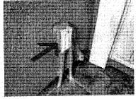
Receptacles are not protected by a Ground Fault Circuit Interrupter (GFCI) at the laundry area, dishwasher, kitchen island counter, wet bar counter, and multiple at the garage interior. The function of a Ground Fault Circuit Interrupter is to protect people from electrical shock hazards. We recommend correction using appropriate methods by a qualified electrical contractor.
