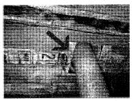
Type B vent piping is cut to make a joint which is improper as viewed at the upstairs heater. Spillage of hazardous exhaust gases can occur as a result, therefore a carbon monoxide poisoning hazard exists. Type B vent piping should utilize factory made snap lock joints. We recommend correction using appropriate methods by a qualified Warm-Air Heating, Ventilating and Air-Conditioning contractor.
