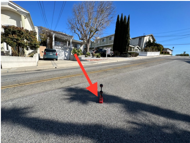
Connection to city sewer under tool.
