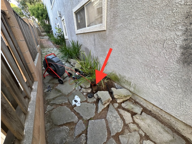
Location of 4" cleanout alongside 1931 ½ used for inspection.
