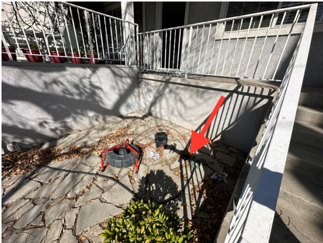
Location of 4" cleanout in front of 1931.
