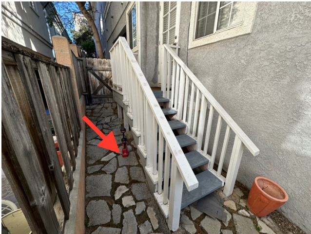
Transition from a cast iron pipe to fiberglass liner.
