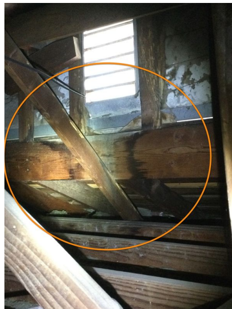
2nd Floor Gable into Attic
