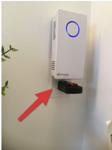
1st Floor Rear Bathroom
