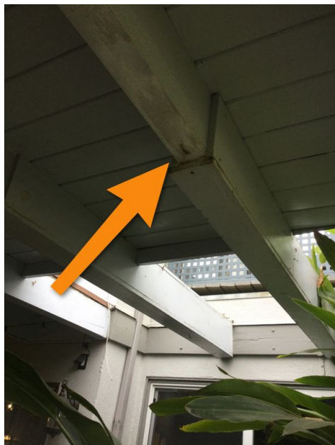
Rear Patio Cover Joists
