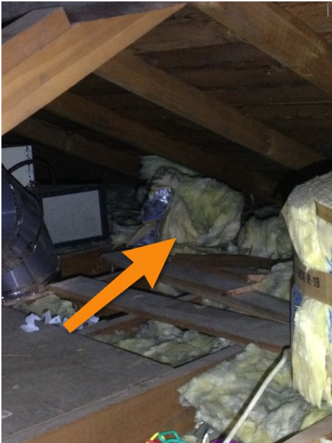
1st Floor Attic
