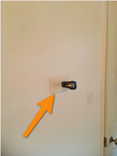
1st Floor Bedroom
