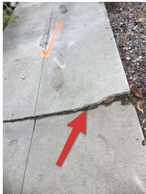
Left Front Exterior
