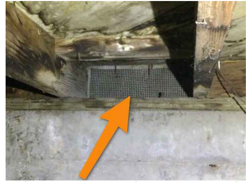
Right Living Room Sub Area-Restricted Ventilation
