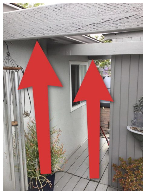
2nd Floor Balcony Cover
