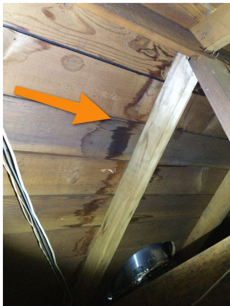
1st Floor Attic
