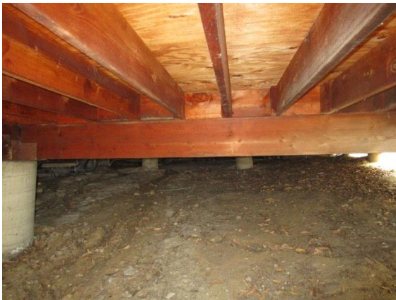
Under Floor Framing & Support:
