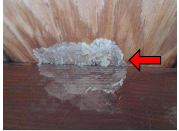
Under Floor Framing & Support:
