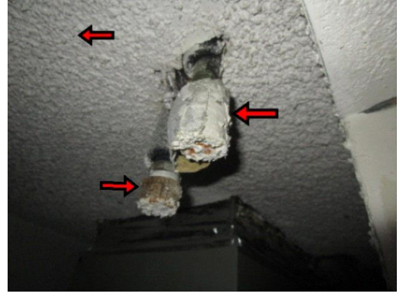
Laundry Facilities: Metal piping and stipple ceiling
