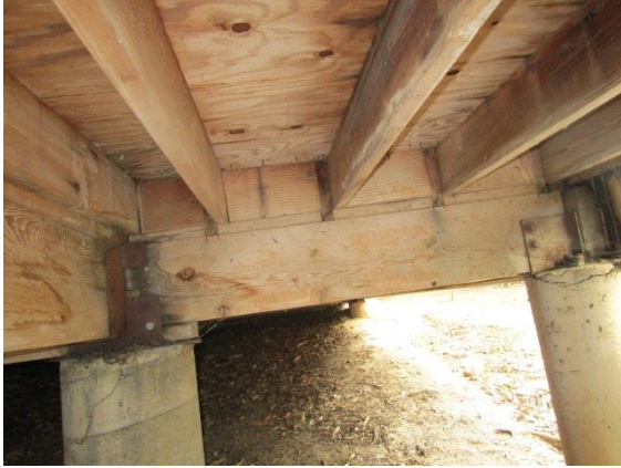
Under Floor Framing & Support:
