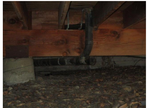
Under Floor Framing & Support:
