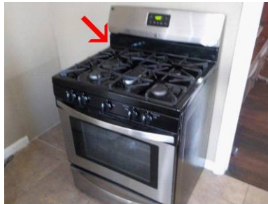
Missing the anti-tip bracket: improper
