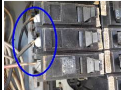
Energized Knob & Tube wiring (hazardous)
