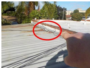
Weather head has inadequate clearance
