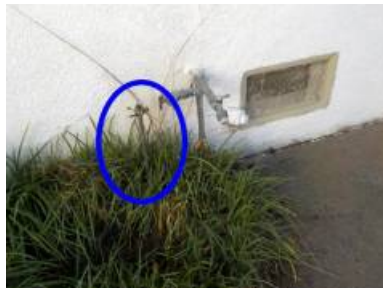
Weather head has inadequate clearance
