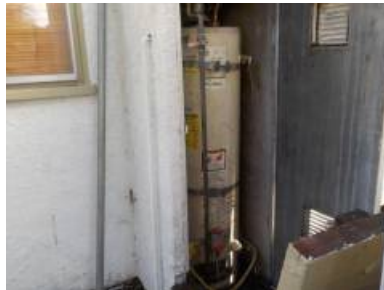
Missing sediment trap/drip leg-improper
