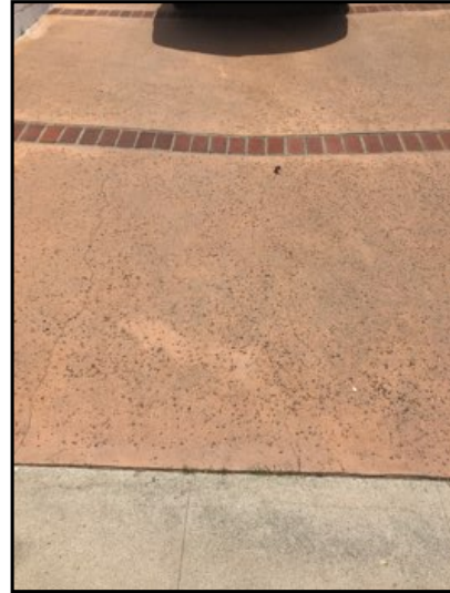
The driveway is in satisfactory condition.
