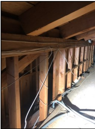
The attic structure is in satisfactory condition.
