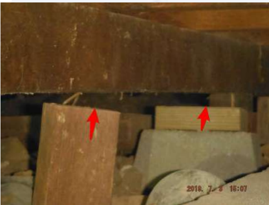
Disconnected posts
