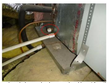
Needs Attention. The secondary drain opening is capped and is not functional.
