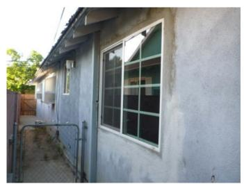
Needs Attention: The stucco has peeling and some deterioration in areas near the level of the soil. There are areas of rough patching, around the windows.
