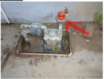
There is an automatic seismic gas shut-off valve installed on the main gas line. It is beyond the scope of this general inspection to determine its operating status or if it has been sized correctly for this gas system. If further information is desired or required it is advised to consult a qualified plumbing contractor.
