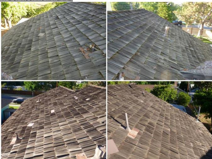
The roofing material on the sloped roof is made of wood shingles.
