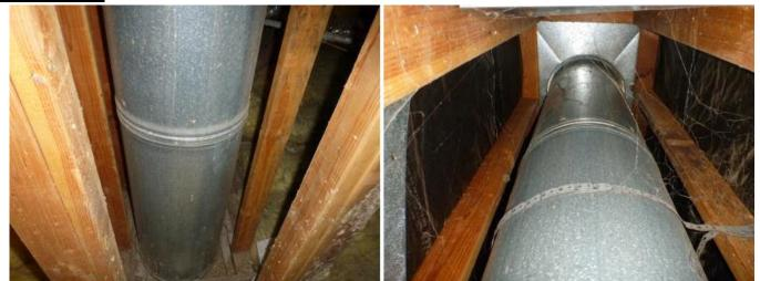
Needs Attention: The flue pipe does not appear to be adequate clearances to combustible materials in the wood framing. It is advisable to have a chimney specialist examine the structure and make all needed repairs to ensure a safe and properly operating fireplace and chimney.
