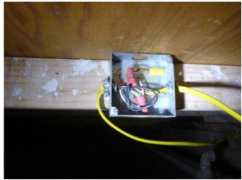
Needs Attention: There are open junction boxes with wires exposed. These need to be completed and have covers installed for safety, in the crawl space under the building.
