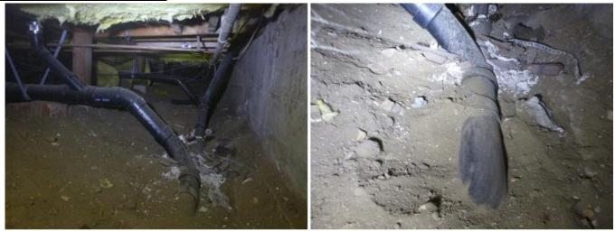
The piping that takes the waste water out to the sewer system has been upgraded with some newer plastic piping in areas but there is still some of the older original lines in use in the system. The older piping that takes the waste water to the sewer system is made of cast iron where visible.
