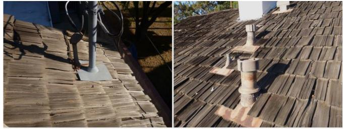
Needs Attention: The flashing is not standard and may not be a reliable installation, such as at the electrical service mast. it will require high maintenance to ensure that it remains leak free.
