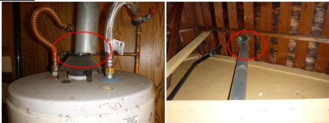
Not Acceptable. The water heater exhaust vent is disconnected, poorly connected or not properly connected. This can allow exhaust gases to escape and is considered a health and safety hazard and should be repaired by a qualified plumber.
