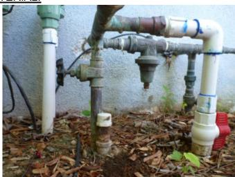
Copper piping is viewed coming out of the ground by the building and as the main line runs underground from the street to the building, this appears to be the main water line. As the underground portion is not seen, no representation is made or implied as to its condition or material.
