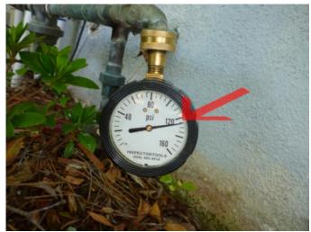
Needs Attention. The pressure is over 80 psi. This is too high, it should be between 40 and 80. The pressure regulator should be adjusted or replaced to bring this down into proper range.
