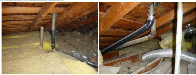
Needs Attention: There are areas of stains on the framing lumber - it is unknown if this is from a current or past roof leak.
