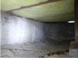
The concrete foundation has some typical cracking, but was in functional condition for a building of this age. Cracking does not appear to be significant at this time. If a more detailed evaluation is required, it could be obtained from a structural engineer or foundation specialist.
