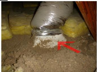
Needs Attention. The insulation of portions the ducts is the type of material that is often found to contain asbestos. It would have to be tested in a laboratory to confirm what its composition is.
