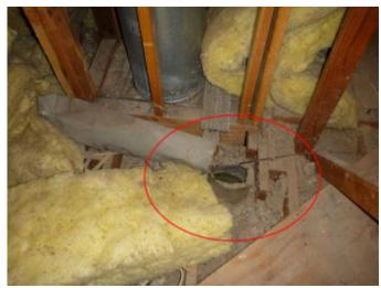
Not Acceptable: The exhaust piping is missing in the attic and this does not vent to the exterior.
