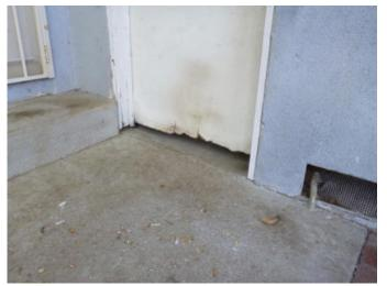
Needs Attention: The exterior side door has areas wear and deterioration to the surfaces.
