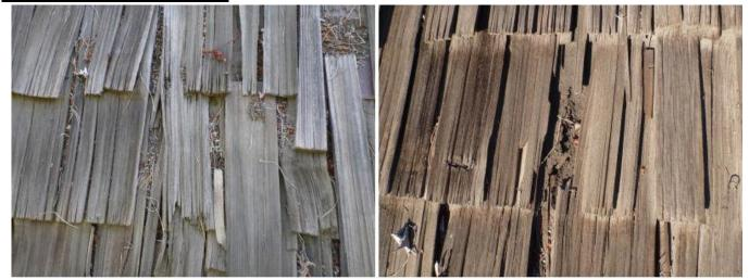
Needs Attention: On the wood roof, the wood shingles are older, warping and deteriorating. They are nearing the end of their life and the time to replace them.
