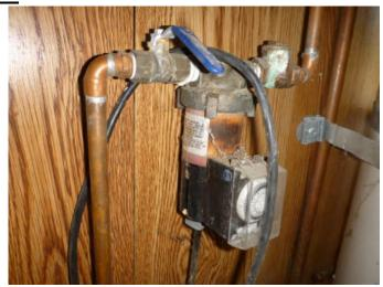
Needs Attention. The re-circulating system was unplugged and off line when it was first located. It was plugged in to see if it would operate but it did not work and was left unplugged.
