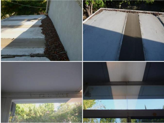
Needs Attention: There is debris on the top of the enclosure, and at the edge drain. There are areas of staining and rusting inside the enclosure below the covering.
