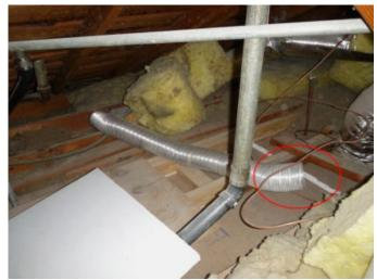
Needs Attention: The ventilation fan in the bathroom does not vent the exterior of the building. The exhaust is going into the attic instead.
