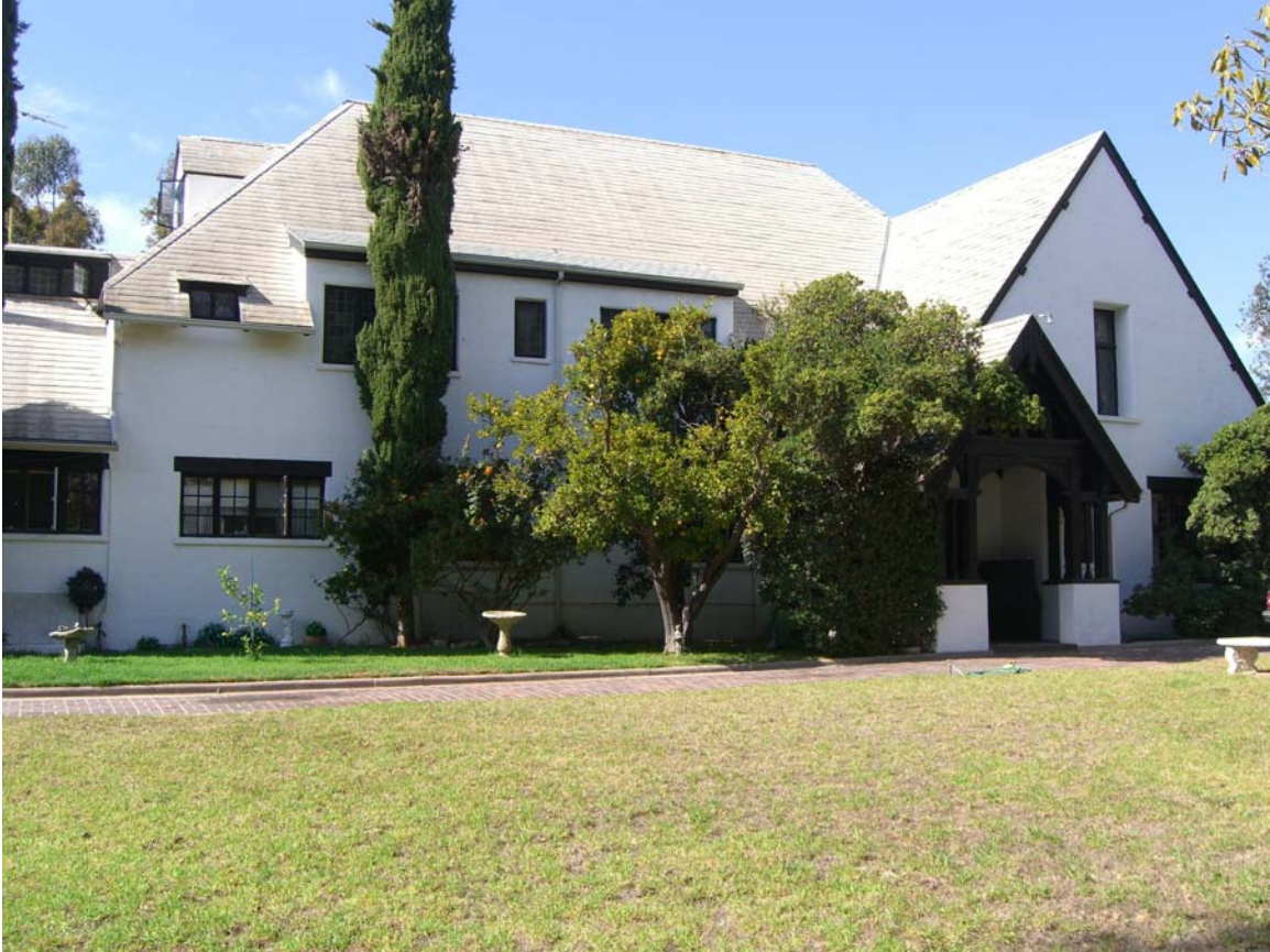
Primary (South Elevation), View North
