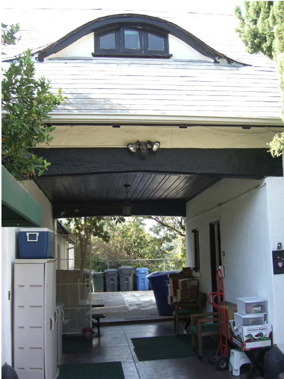
Porte-Cochere, View North
