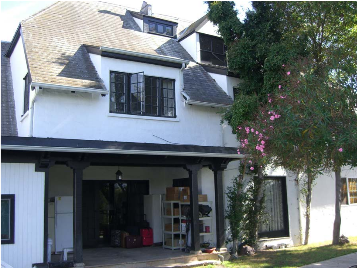
North Elevation, View Southwest
