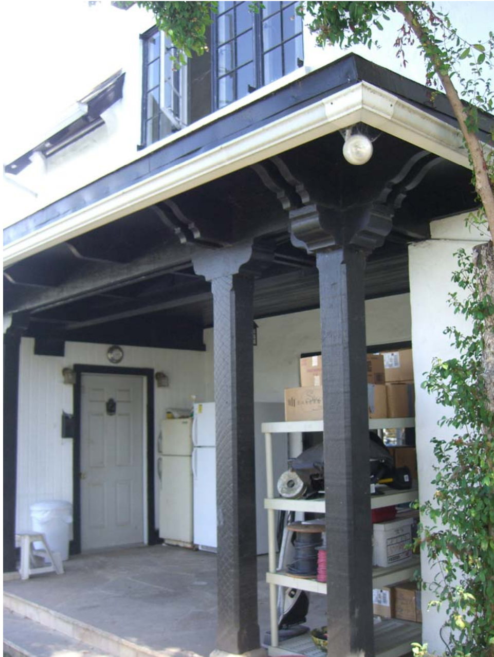
North Elevation, View Southeast
