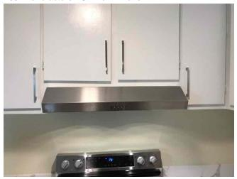
**161:** Kitchen ventilation is provided by a range hood over the burners. The fan appears to be properly installed and in serviceable condition.
