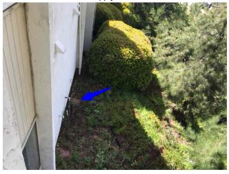
**4:** The main shut-off valve was not located and it is possible that there is no shut-off valve for only this unit. Information regarding this matter should be available from the homeowner's association.
