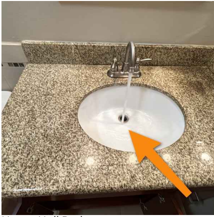
Upper Hall Bathroom
