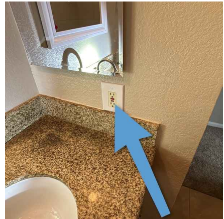
Upper Hall Bathroom
