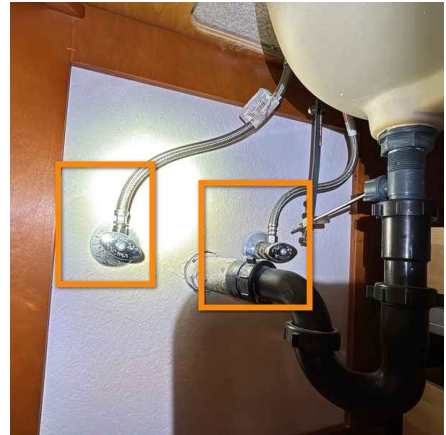
Upper Hall Bathroom
