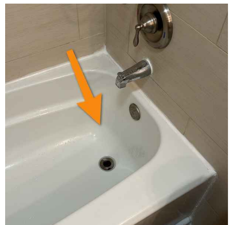
Upper Hall Bathroom
