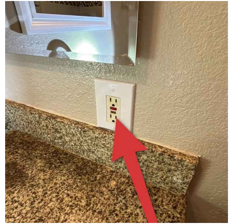
Upper Hall Bathroom
