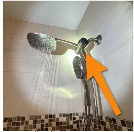
Upper Hall Bathroom
