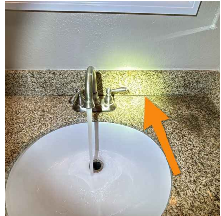
Upper Hall Bathroom
