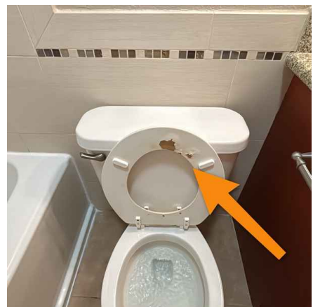
Upper Hall Bathroom
