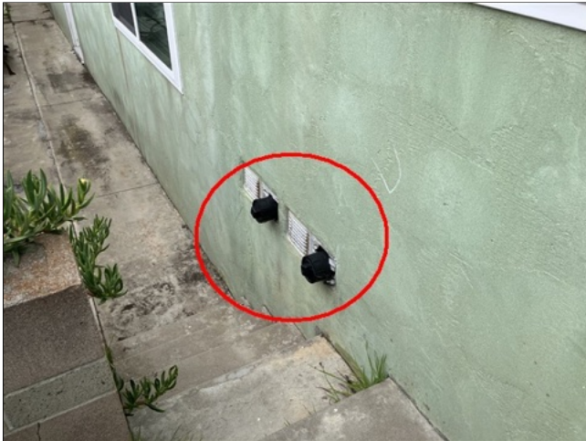
6.3 Item 3(Picture) sewer camera inspection recommended
