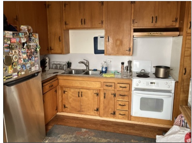
4.8 Item 10(Picture) unit 4772 kitchen
