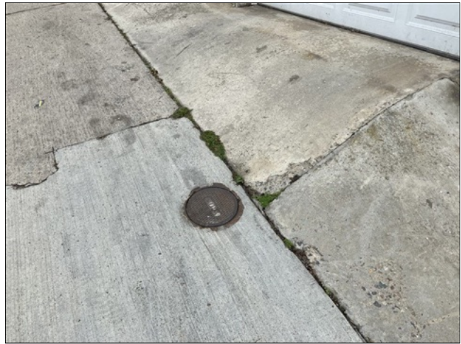
6.3 Item 2(Picture) sewer camera inspection recommended
