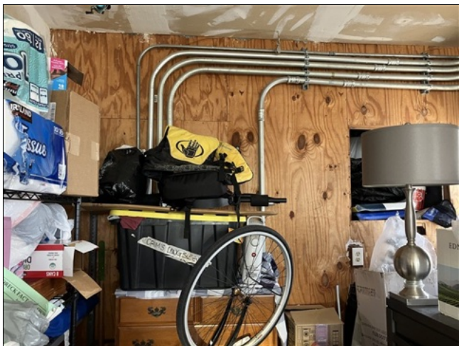
3.1 Item 3(Picture) unit 4772 garage: firewall upgrades recommended
