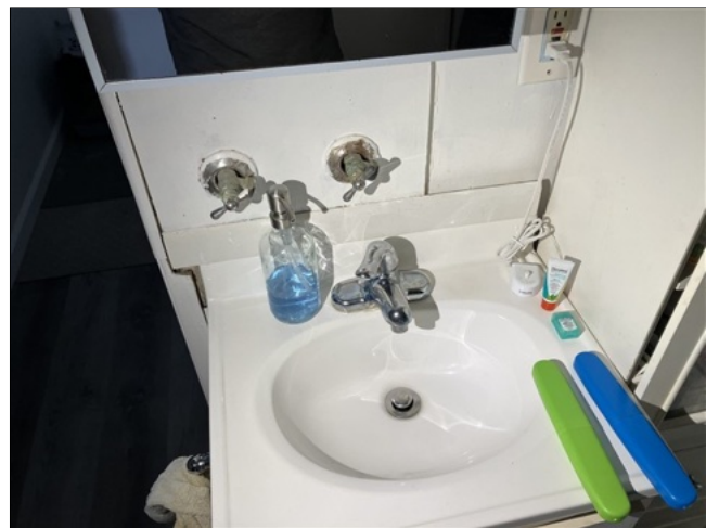
4.8 Item 8(Picture) unit 4770: bathroom #2 appeared to be an addition
