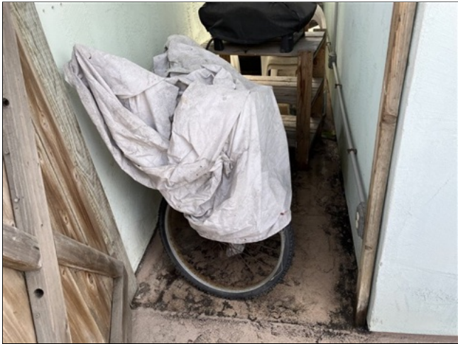
2.6 Item 4(Picture) limited access and/or visibility
