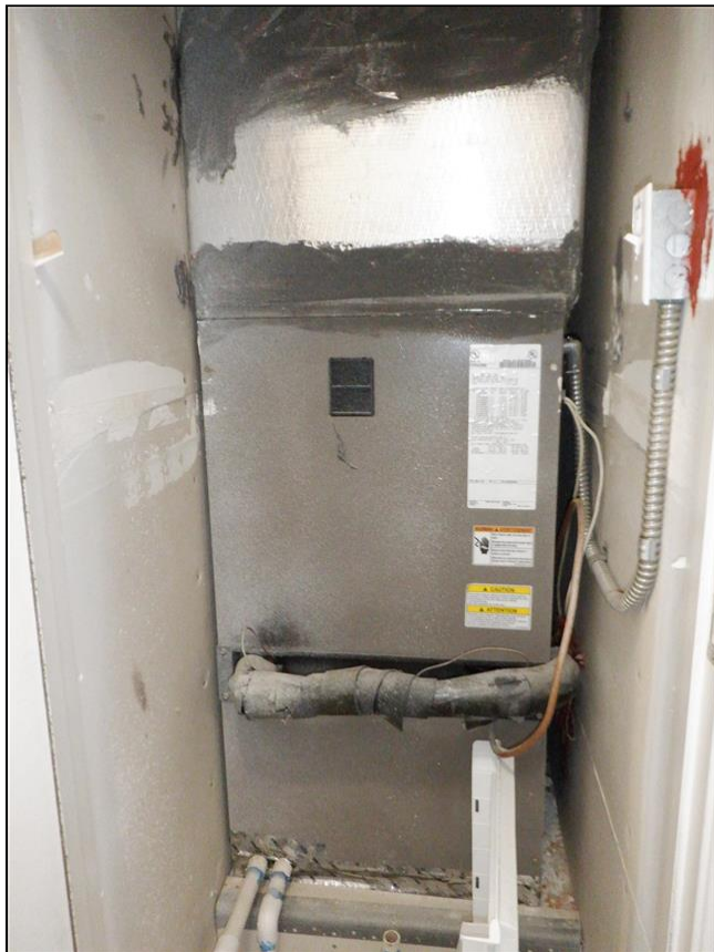
9.0 Item 1(Picture) Electric heat pump
