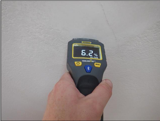
4.0 Item 1(Picture) Moisture test at living room ceiling repair
