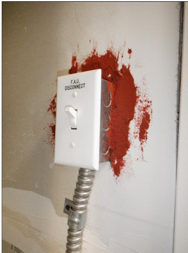
9.0 Item 2(Picture) Power switch for heat pump
