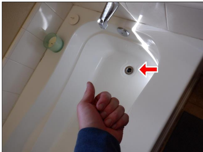
5.5 Item 10(Picture) Tub drains properly
