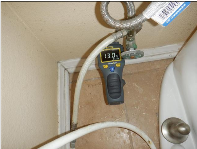
5.1 Item 5(Picture) Moisture test around plumbing fixtures
