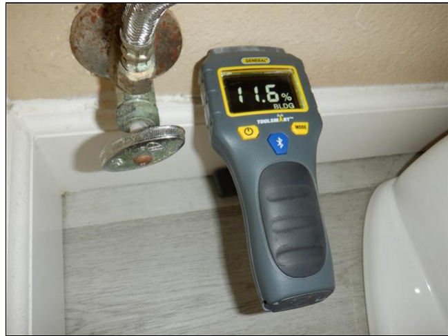
5.1 Item 4(Picture) Moisture test around plumbing fixtures
