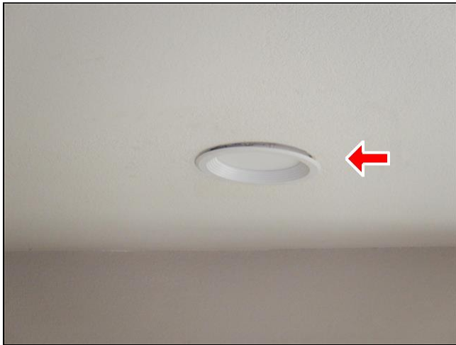
4.6 Item 3(Picture) Loose an light at entry
