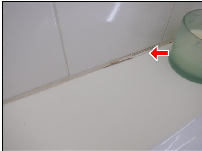
5.4 Item 2(Picture) Worn grout
