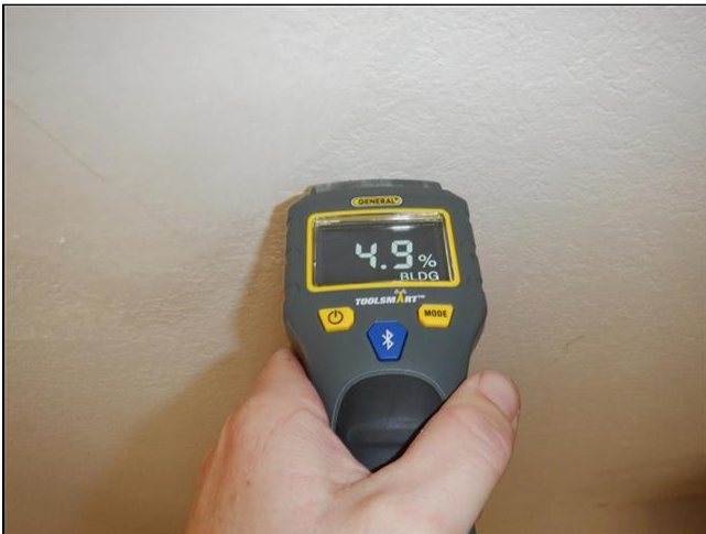
4.0 Item 3(Picture) Moisture test at living room ceiling repair
