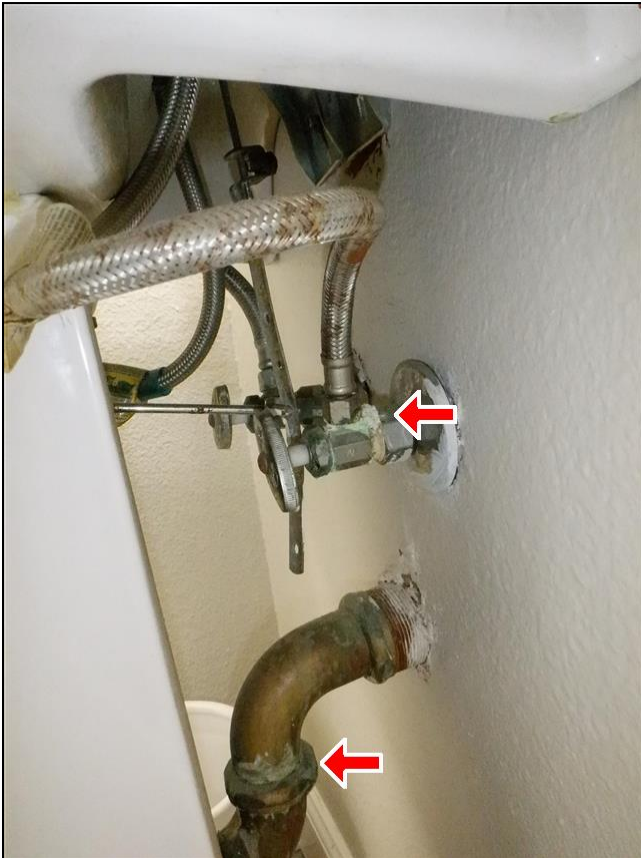
5.5 Item 1(Picture) Corrosion at pedestal sink
