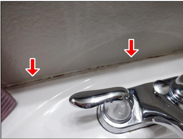
5.4 Item 1(Picture) Pedestal sink not sealed
