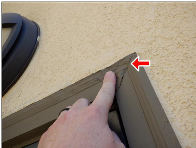
2.1 Item 2(Picture) Soft trim on water heater closet door
