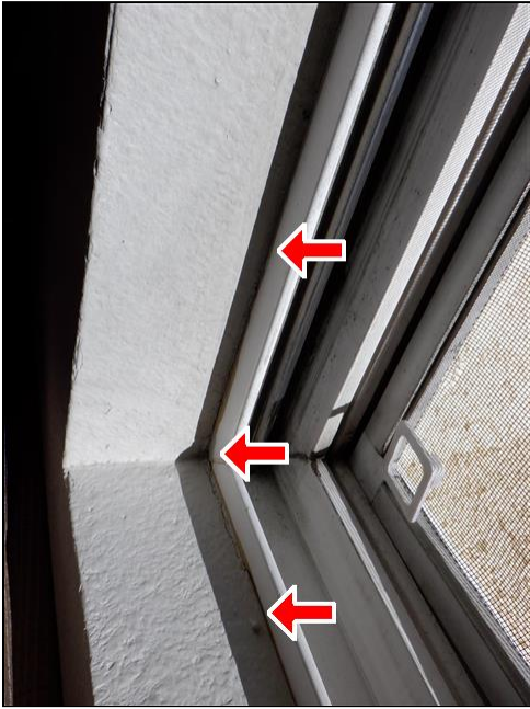
4.5 Item 1(Picture) Cracking in window sills
