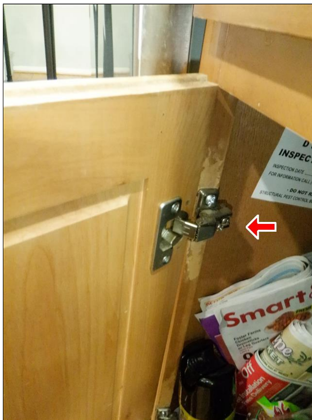
3.3 Item 2(Picture) Loose cabinet hinges
