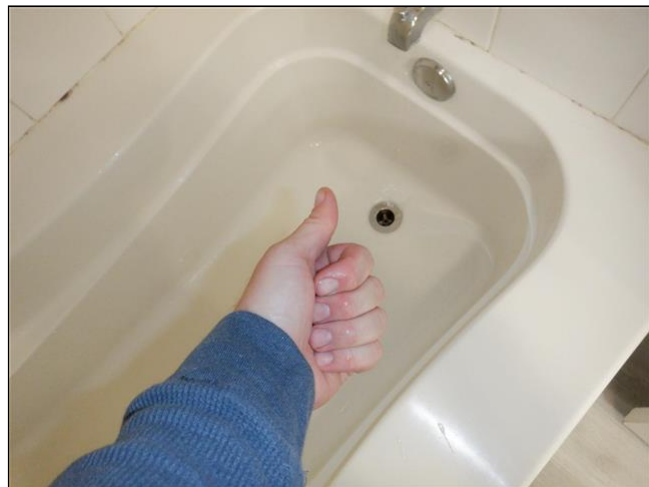
5.5 Item 6(Picture) Tub drains properly
