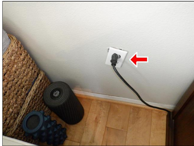
4.6 Item 4(Picture) Loose receptacle cover plate
