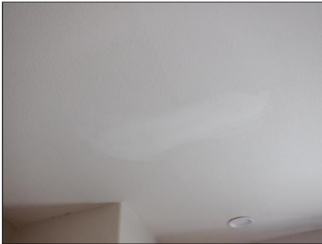
3.0 Item 1(Picture) Repair to ceiling
