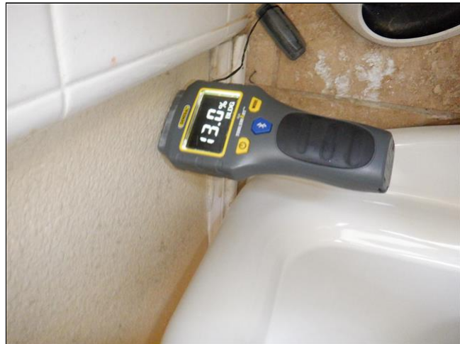
5.1 Item 6(Picture) Moisture test around plumbing fixtures
