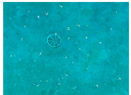
Flat covers are older in design and can cause entrapment due to the vacuum that is created
