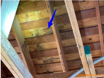
Water stains on newer sheathing
