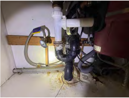
P-trap could leak again any anytime
