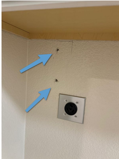
Example Laundry room
