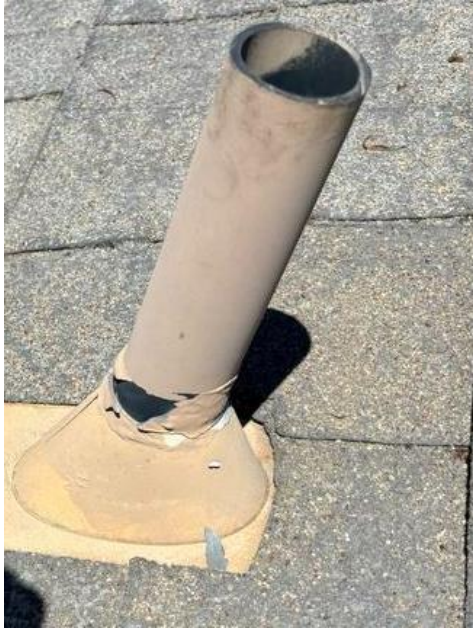
Examples of pipes need sealing
