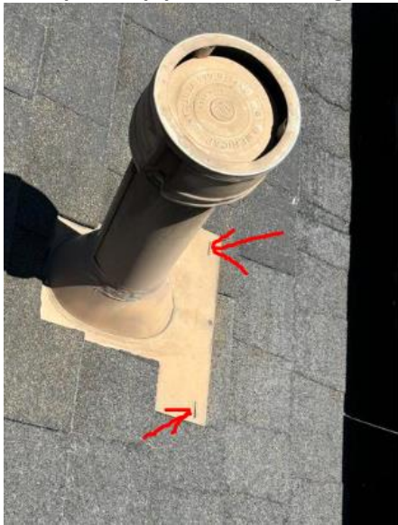
Examples of exposed fasteners
