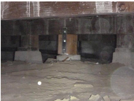
Under Floor Framing & Support:
