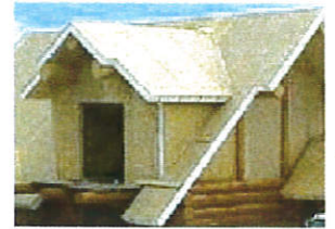
SIP Walls and Roof
