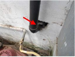
➤ Cast iron drain lines have limited service life and tend to corrode and scale on the inside, which in turn causes the drains to run slowly. Determining the condition of the interior of the drain lines requires specialized equipment and is beyond the scope of this inspection. It is recommended that a licensed plumbing contractor having closed circuit television capabilities be retained in order to determine the condition of the interior of the drain lines.
