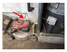
➤ There is no water heater expansion tank installed. Most local jurisdictions require an expansion tank to limit pressure buildup in the water supply system.
