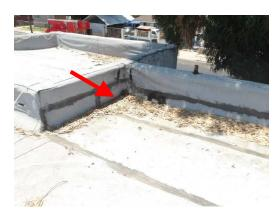
➤ There are wrinkles in the roofing in places. This condition is caused by incomplete bonding of the roofing plys.
