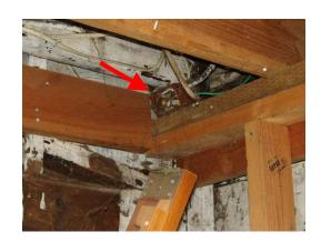
➤ The electrical conduit between the garage and house is damaged and this wiring is in need of repair.
