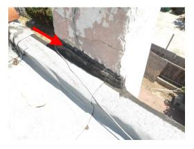
➤ The eaves at deteriorated at the northeast portion of the house. It is recommended that a licensed structural pest control company be contacted for further inspection and repair recommendations.
