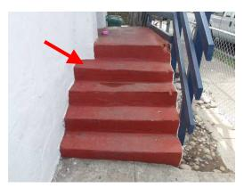
➤ The exterior stairways at the north and south sides of the building should be provided with handrails as required by local building codes.
