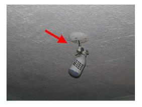
The homes are equipped with smoke alarms in the hallway and kitchen of 219 South 29<sup>th</sup> Street and in the hallway of 221 south 29<sup>th</sup> Street. The smoke alarm in the hallway of 219 South 29th Street sounded when the "test" button was pressed. The Client is
