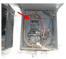
The main electrical sub-panel is located outside at the southwest corner of the garage. Overload protection is provided by circuit breakers. The wires visible in the sub-panel are copper.
