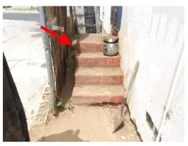
> The entry stairway railing is sound, however, the railing is not of a readily "graspable" type. Current local building codes require that railings be of a "graspable" type, however, this may have not been required at the time of construction.
