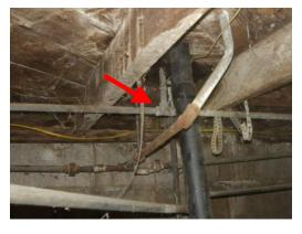
inspection if all portions of the galvanized steel piping, particularly those portions inside the walls, have been replaced. It is recommended that a licensed plumbing contractor be contacted for further inspection of the water supply system and for recommendations.
