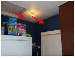
➤ The damaged and patched areas are apparently the result of roof leakage. Water intrusion can cause damage to the structure, as well as promote the growth of mold and mildew. It is beyond the scope of this inspection to determine the presence of potentially harmful mold and mildew. It is recommended that a qualified indoor air quality specialist be contacted for comprehensive investigation and for recommendations.
