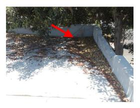
➤ The roof drain downspouts discharge adjacent to the foundation and should be reconfigured to drain away from the foundation.
