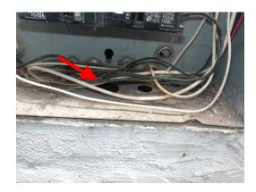
➤ The capacity of the wires feeding the panel are only 30 amps, however, the breaker feeding the panel appears to be 40 amps. This condition should be corrected.
