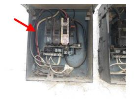
➤ One of the left panel breakers is of the Federal Pacific "Stab-Lok" type. This type of breaker has been shown to be a hazard in some cases.
