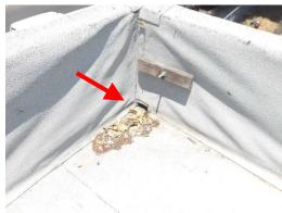
➤ There is debris present on the surface of the roof. The roof should be cleared of debris.
