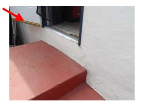
The front doors do not seal tight and are in need of adjustment or repair.
