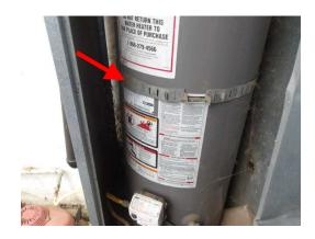
The right water heater outside at the rear of the house is a gas fired Rheem model with a 40 gallon storage capacity. The gas vent is serviceable at this time. The gas supply shut-off valve is properly installed and no smell of gas was detected. The water supply shut-off valve and pressure-temperature relief valve are also properly installed. The pressure-temperature relief valve is vented to the ground. The water heater is secured by seismic restraints.
