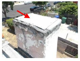
> The chimney may not have a tile liner and may be subject to earthquake damage. This condition can also cause the chimney to become unsafe for burning solid fuels.
