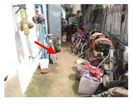
line, the soil may slope at the same rate to a swale which drains to the street or to another proper drainage discharge area. In correcting the drainage care must be taken to keep the soil level a minimum of 6 inches below the top of the foundation wall to prevent possible moisture intrusion into the wall assembly and deterioration of the wood framing.
