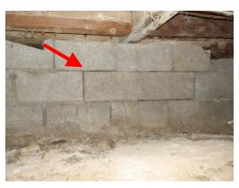
➤ The east foundation wall has gaps between the blocks in places. This condition is also apparently caused by some movement of the foundation.
