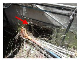
Some of the posts consist of stacked blocks and there may not be concrete piers for these posts. All posts should be continuous and provided with piers for support.
