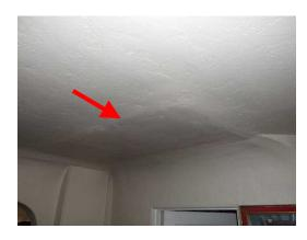
The ceiling in the bathroom is sagging. This condition is possibly the result of roof leakage. It could not be determined by visual inspection if this condition is caused by on-going leakage or if the leakage has been repaired.
