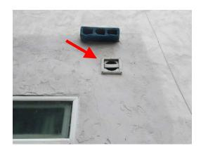
➤ There is a joint in the stucco at the main house/addition junction. This condition is apparently caused by some differential movement between the main house and the addition.
