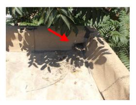
> The roof drain downspout at the northeast corner of the garage is missing and should be replaced.
