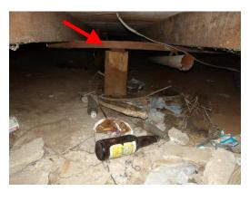
➤ There is some deterioration to the wood framing, especially near the north most access hatch. It is recommended that a licensed structural pest control company be contacted for further inspection and repair recommendations.
