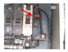
➤ The capacity of the main breaker for the right panel is only 40 amps. The Client should be aware that this may not be sufficient for modern day appliances or for adding circuits.
