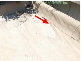
➤ There are no secondary roof drains present. Current local building codes require secondary roof drains. This may not have been required at the time of construction.
