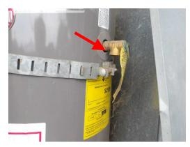
➤ The water heater is secured by seismic restraints, however, the lower restraint is too high and should be relocated to the lower 1/3 of the water heater.
