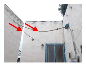
There is a disconnect outside at the rear of the house which is being used as a junction box. This box should be sealed shut.
