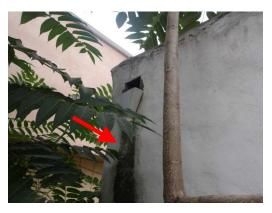
The roof drain downspout at the west side of the house discharges to the area around the foundation and should discharge away from the foundation.
