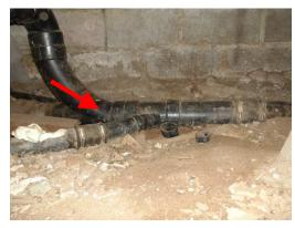
> The plumbing vent outside at the rear of the building left of the water heaters is disconnected and is in need of repair.
