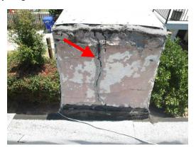
➤ The to the chimney has been capped off. The cause for this condition was not determined.
