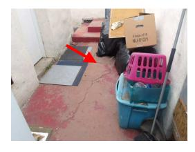
➤ There is evidence of water ponding on the patio at the east side of the house. The drainage should be improved in this area and water should not be allowed to pond in areas adjacent to the foundation.
