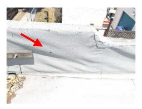
➤ There are no secondary roof drains present. Current local building codes require secondary roof drains. This may not have been required at the time of construction.
