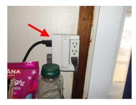
Current local building codes require that ground fault circuit interrupt (GFCI) protection be provided for certain interior and exterior electrical outlets. A GFCI breaker is a safety device designed to help prevent injury which may be caused by faulty electrical appliances or by accidental contact with energized circuit components. GFCI protection was not required for homes built before approximately 1973 and does not appear to have been required at the time of construction.
