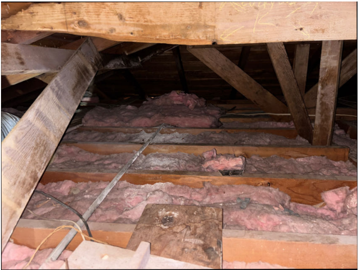
Framing- Conventional rafter type framing present.
