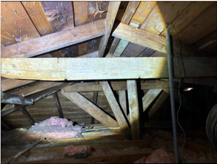
Framing- Conventional rafter type framing present.
