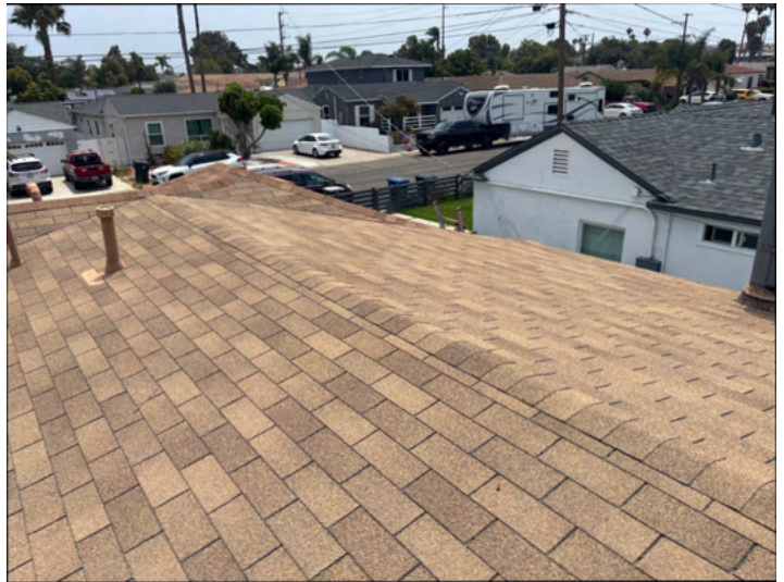
Picture of the composition shingle roof.
