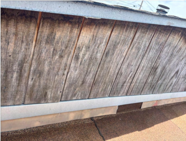
The overall condition of the wood siding's paint is fair as sections may require additional paint, paint touch up and or service. Location: Rear of the home at the gable end.
