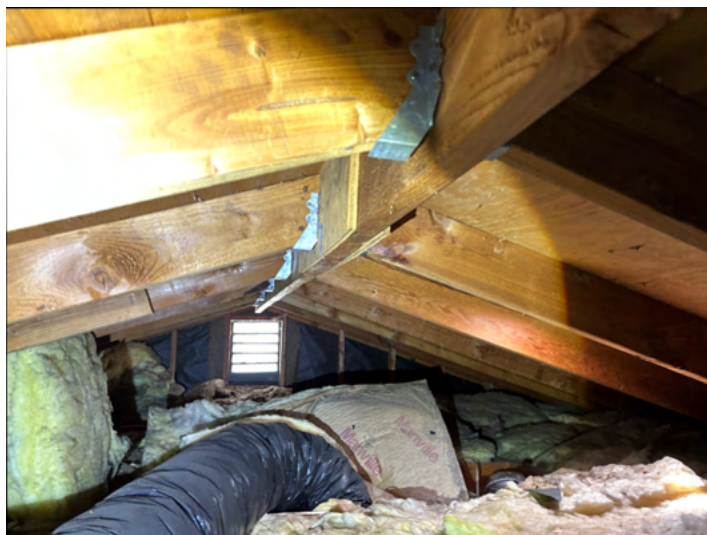
Framing- Conventional rafter type framing present.
