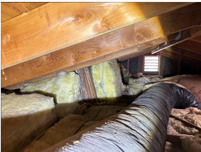
Framing- Conventional rafter type framing present.
