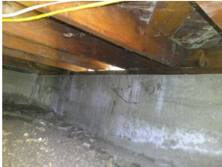
Picture of the raised foundation exterior walls.
