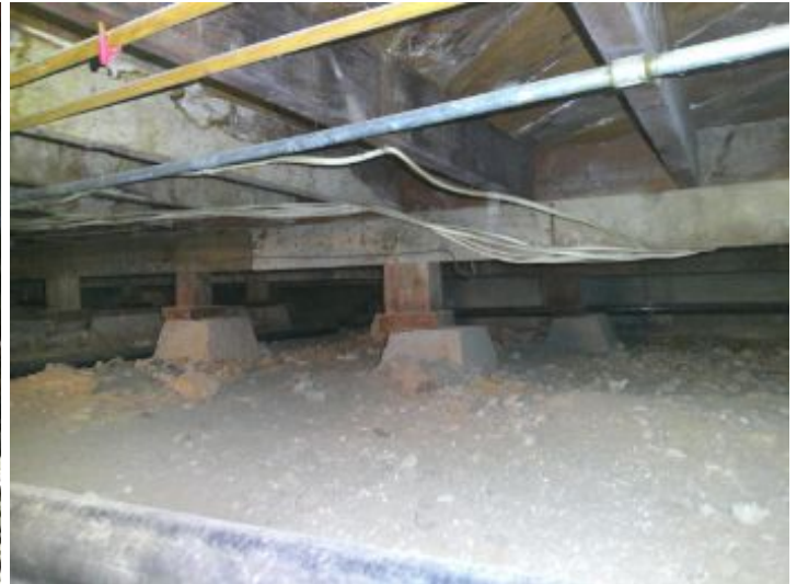
Picture of the floor framing.
