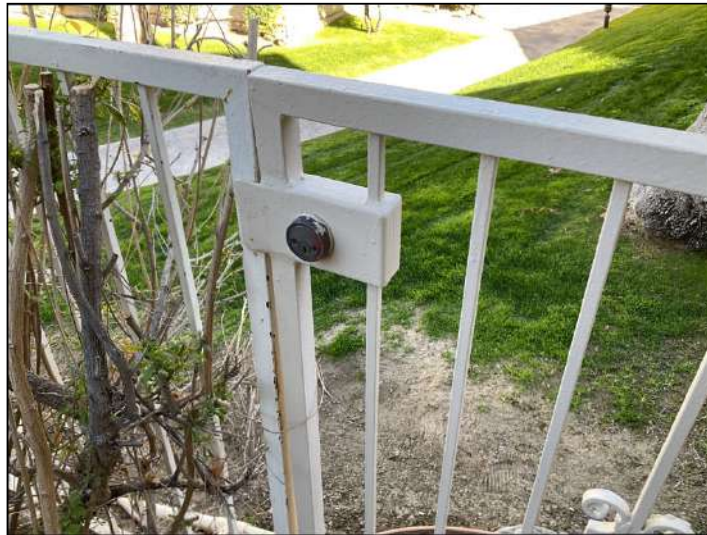
Gate was locked at the time of inspection, did not test.
