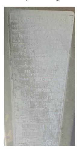
The date of production/manufacture or age of Bryant brand HVAC equipment can be determined from the serial number located on the rating data plate.
