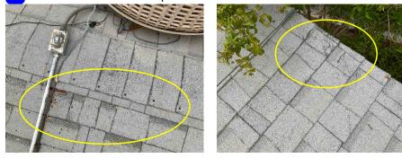
**NR 4:** Nails/Fasteners are protruding from the roof surface. Recommend the entire roof be evaluated and repaired by a qualified Roofing Contractor
