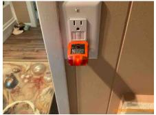
**SC** 33: Receptacle in bathroom is not grounded and protected by a GFCI receptacle, GFCI protected receptacles are required in all bathrooms, Recommend further review and repairs as needed by a Qualified, State Licensed Electrical Contractor.
