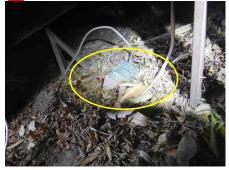
**SC** 35: Loose junction box and conduit with exposed wiring noted. Recommend further review and repair by qualified Electrical Contractor.
