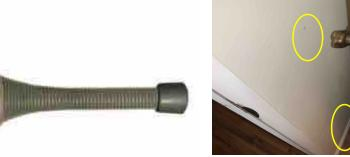
**50:** Door stop is missing, recommend installation of door stop to prevent damage to bathtub
