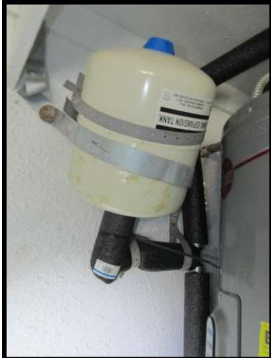
Improperly Mounted Expansion Tank noted
