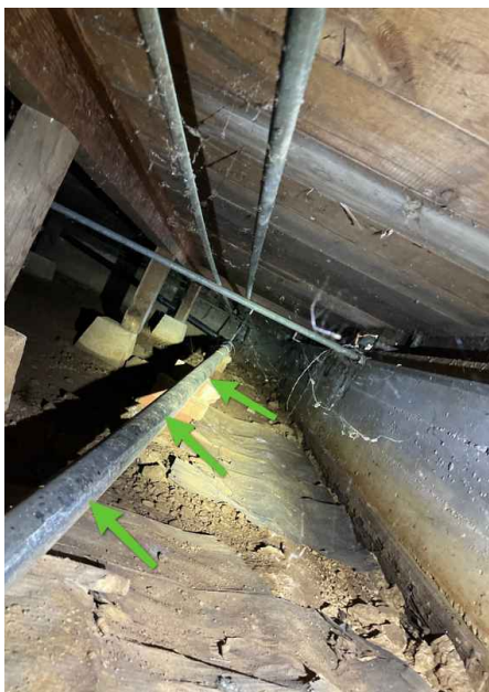
Some of the drain lines had been replaced with new ABS pipe
