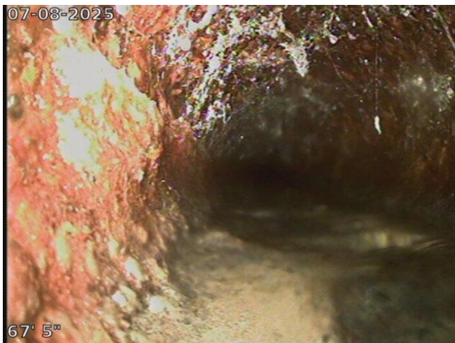
2025-07-08-10-17-30.mp4-thumb Scale buildup in the Cast Iron / The furthest point the camera could go from the toilet sweep on the left side of the house
