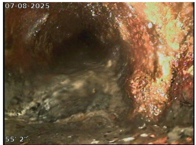
2025-07-08-10-18-18 Scale buildup in the Cast Iron
