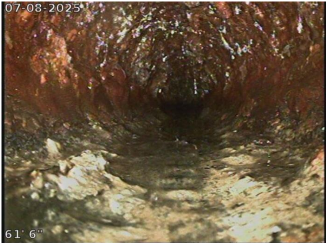
2025-07-08-09-54-04 Scale buildup in the Cast Iron
