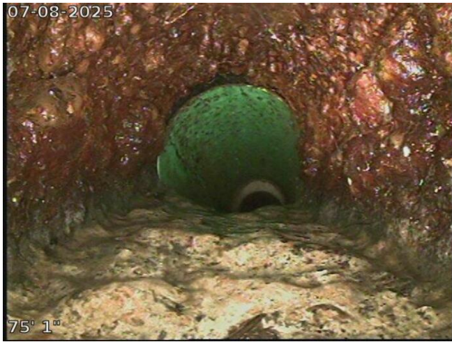
2025-07-08-09-53-32 Cast Iron to PVC connection
