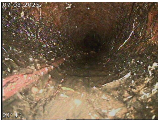
2025-07-08-09-55-32 Damaged Cast Iron
