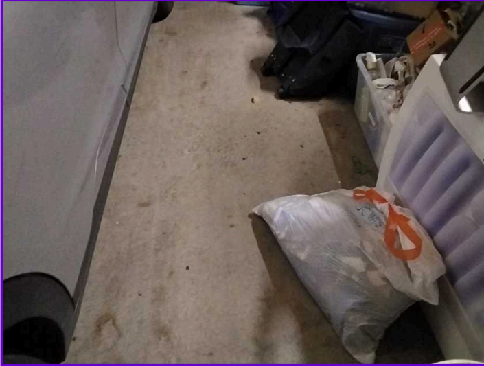
Garage Foundation Concrete Slab
