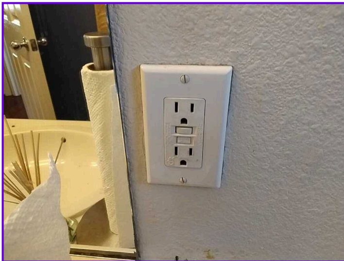
GFCI Protection GFCI Receptacle Outlets
