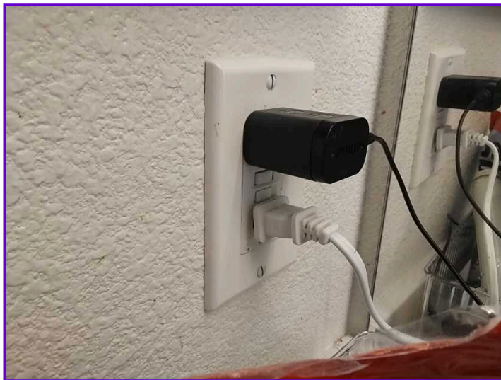
GFCI Protection GFCI Receptacle Outlets
