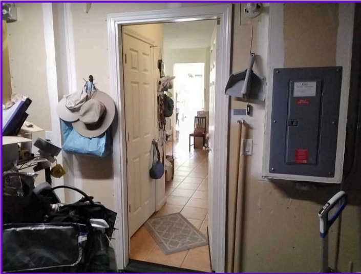
Garage Interior Fire Door
