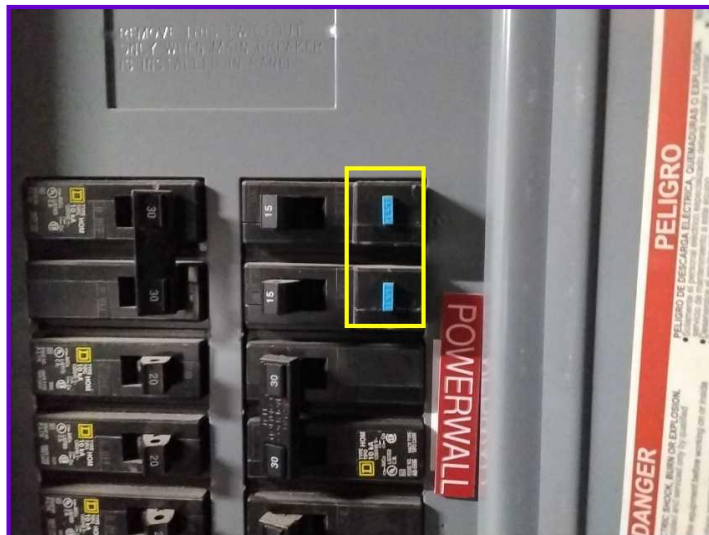
AFCI Protection AFCI Breakers
