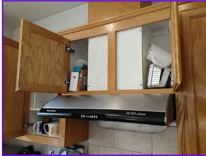
Ventilation and Exhaust Kitchen
