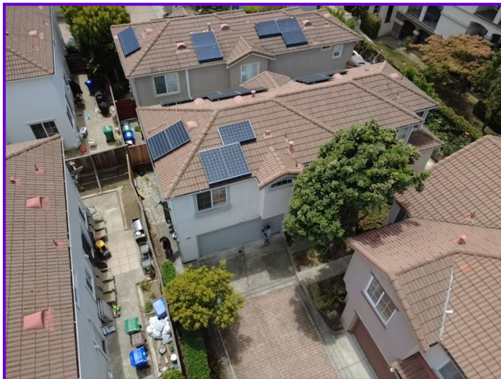
Primary Roof General Comments
