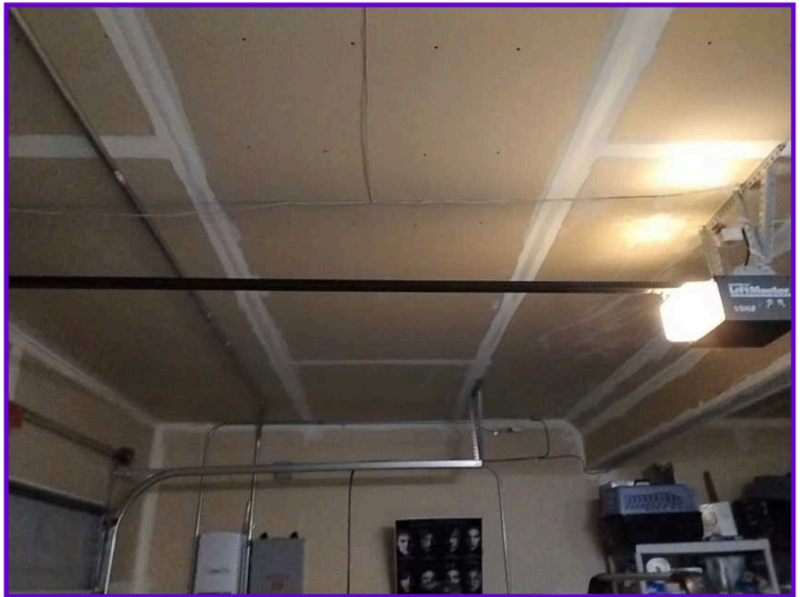
Garage Interior Walls and Ceiling
