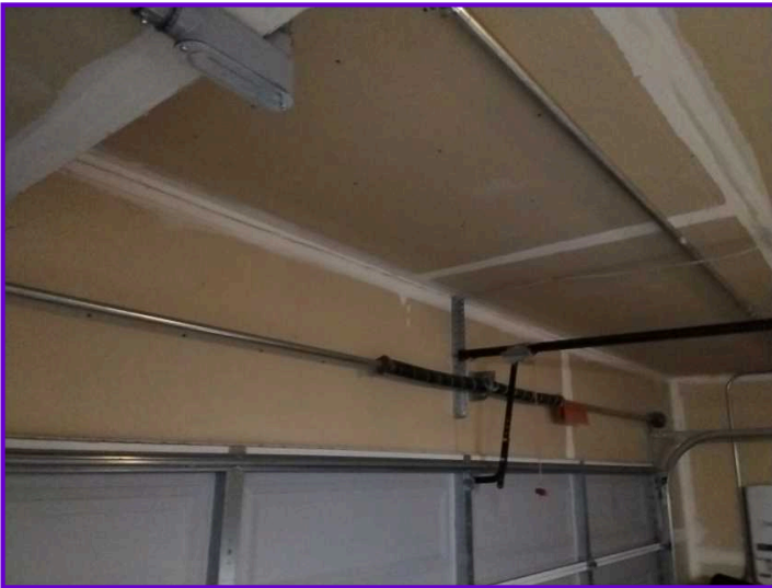
Garage Interior Walls and Ceiling
