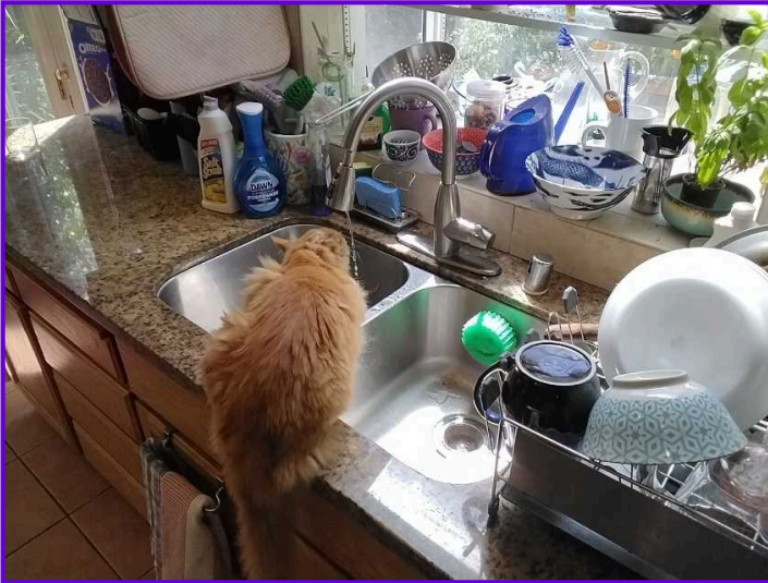
Plumbing Fixtures Sinks
