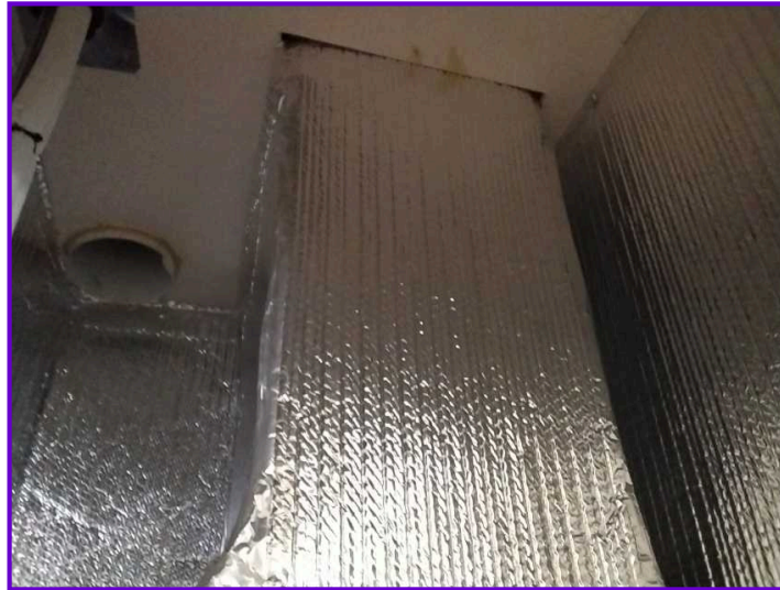
Heat Pump Heat and AC
