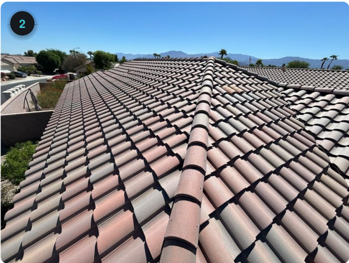
Figure 2 — Roof overview, hip & ridge line No widespread deterioration observed
