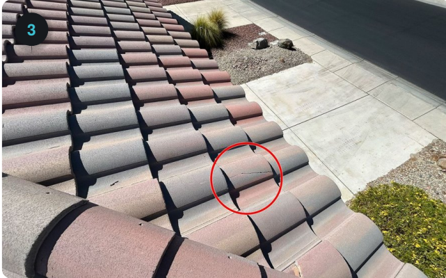
Figure 3 — Chipped tile, eave-line view
