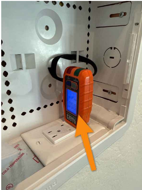
Example Noted At Living Room
