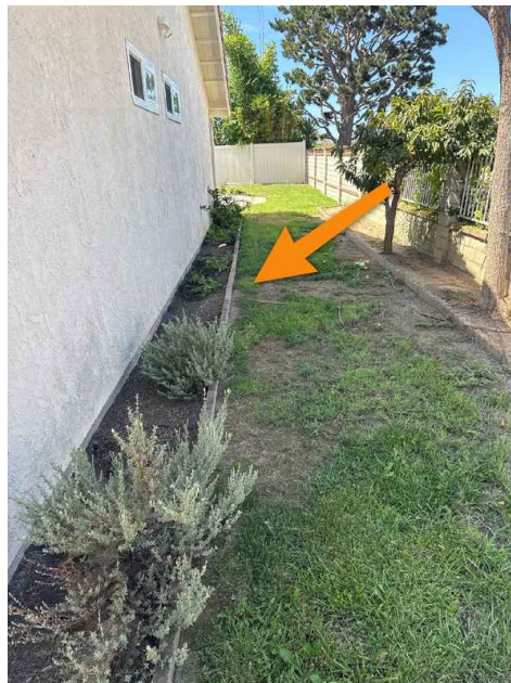
Example Noted At Right Side Of Home
