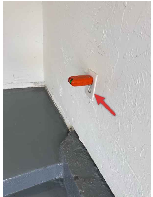
Example Noted At Garage
