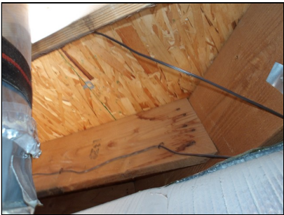
master bedroom attic
