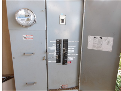
Electric front exterior
