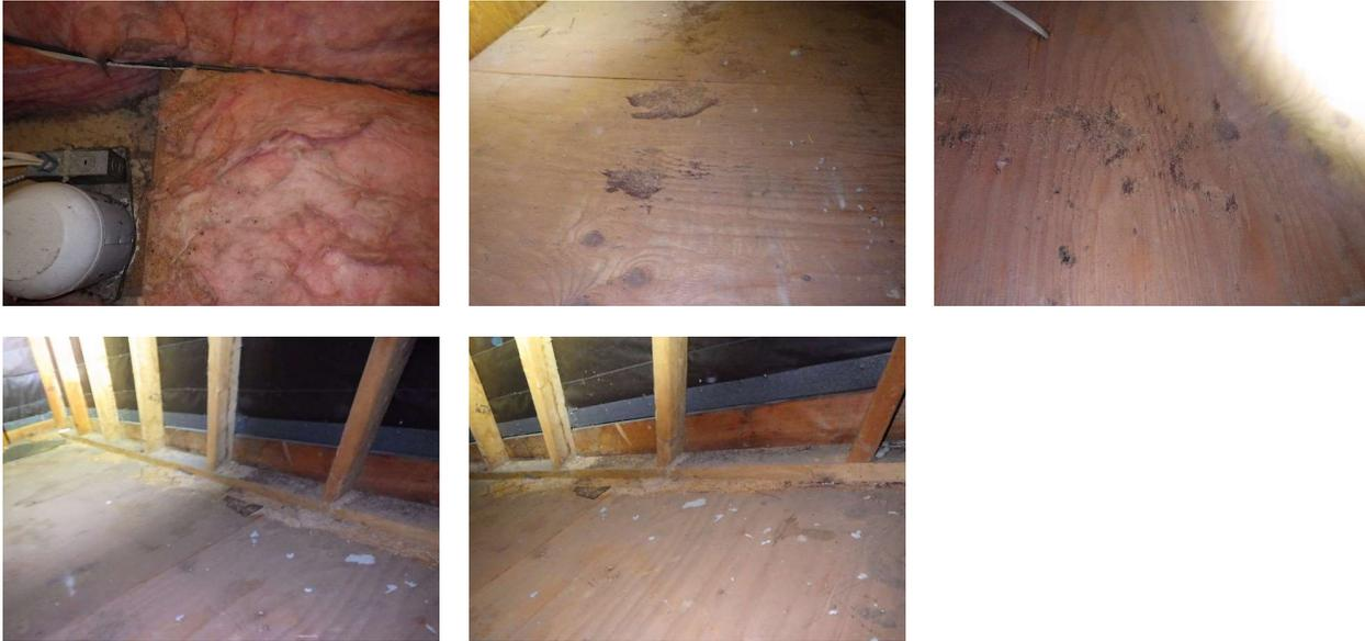
16.5 - There is evidence that the roof has leaked in several locations, which should be reasonably explained, or the roof should be further evaluated by a licensed roofer.
