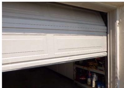
15.14 - The weather stripping is damaged and or missing on the bottom of the door, which should be repaired or replaced.
