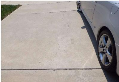
2.19 - There is an offset at the intersection of the driveway and garage slab, which may pose as a trip hazard and may indicate movement has occurred. Further evaluation and repair by a licensed foundation contractor is advised.
